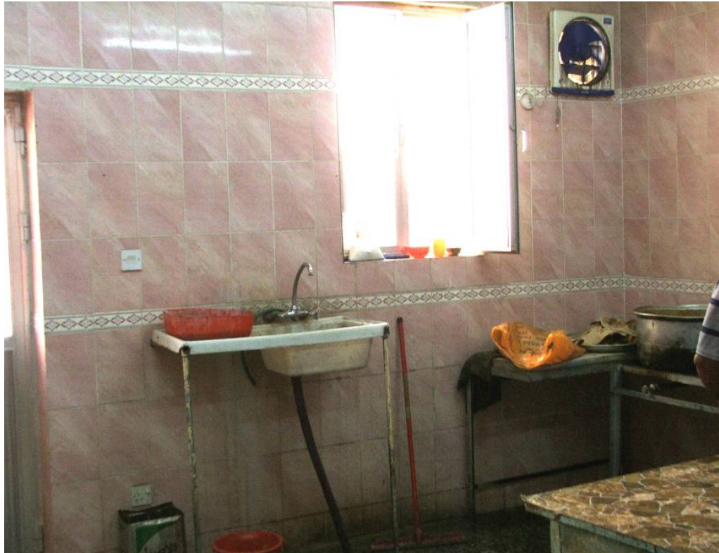
Site Photo 7. Interior of Kitchen Area
