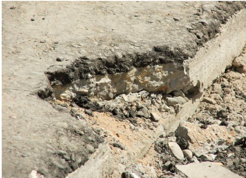
Site Photo 10. Edge of Helicopter Pad
