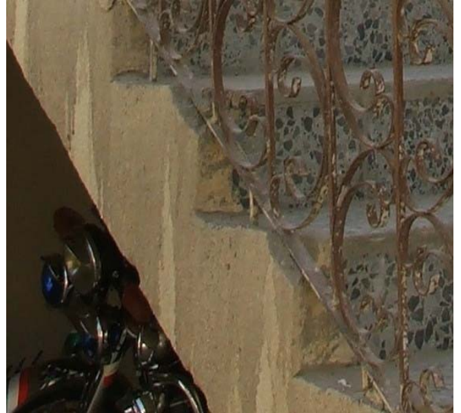
Site Photo 3. Close-Up of Stairwell
