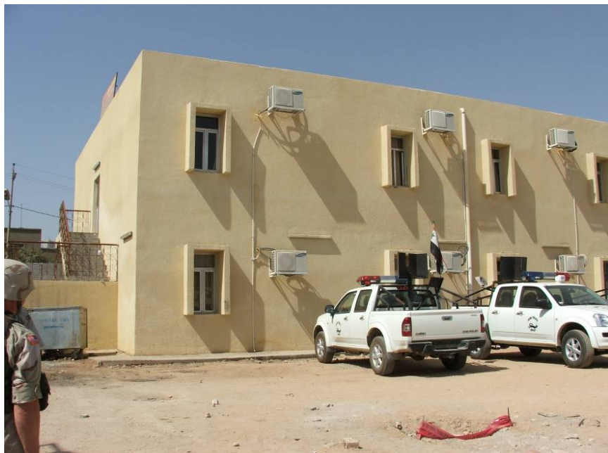
Site Photo 1. Exterior Front of Two-Story Sleeping Quarters Building
