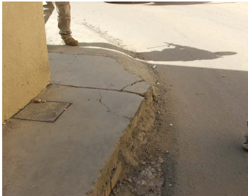
Site Photo 15. Sidewalk of Vehicle Affairs Building
