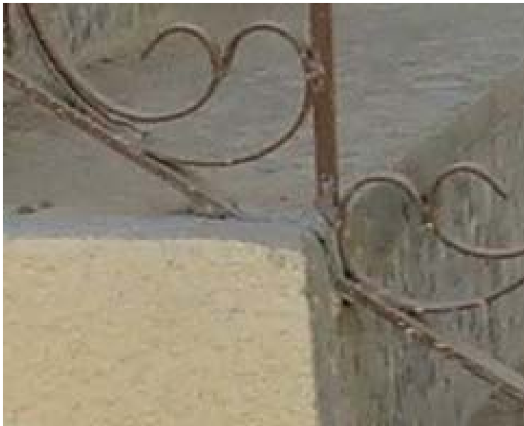
Site Photo 13. Lower Stairwell Railing of Operations Room
