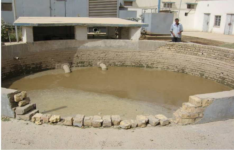
Site Photo 8: Sludge tank
