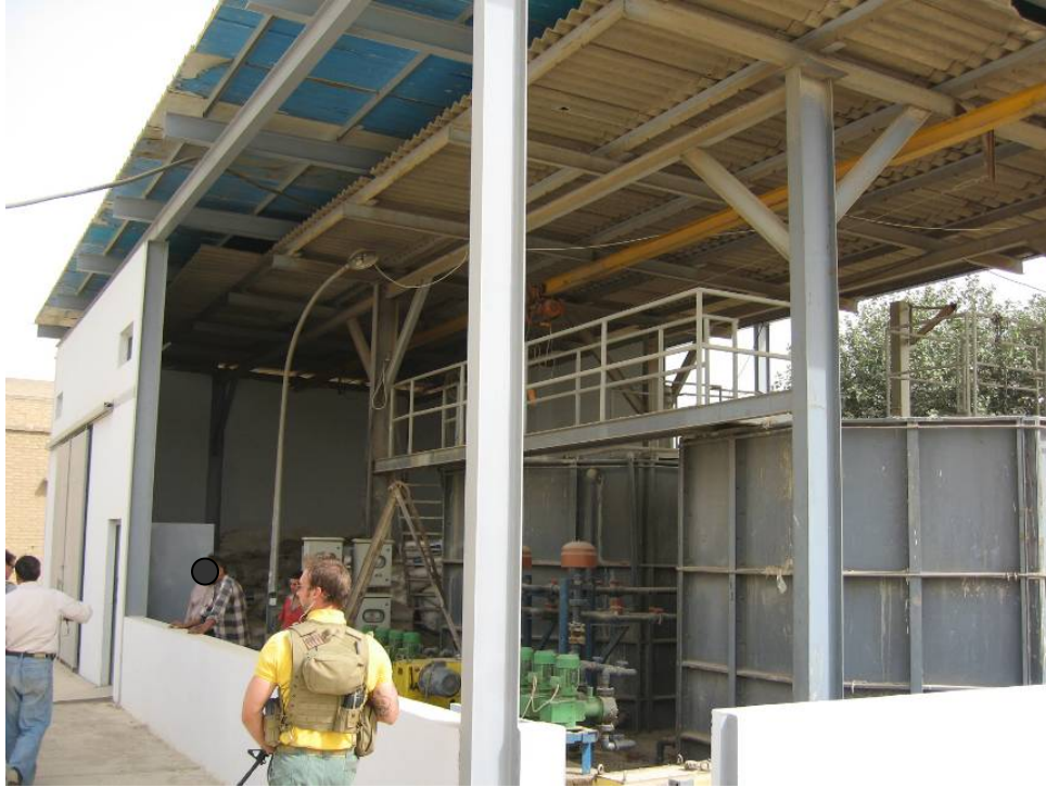
Site Photo 4: New chemical building
