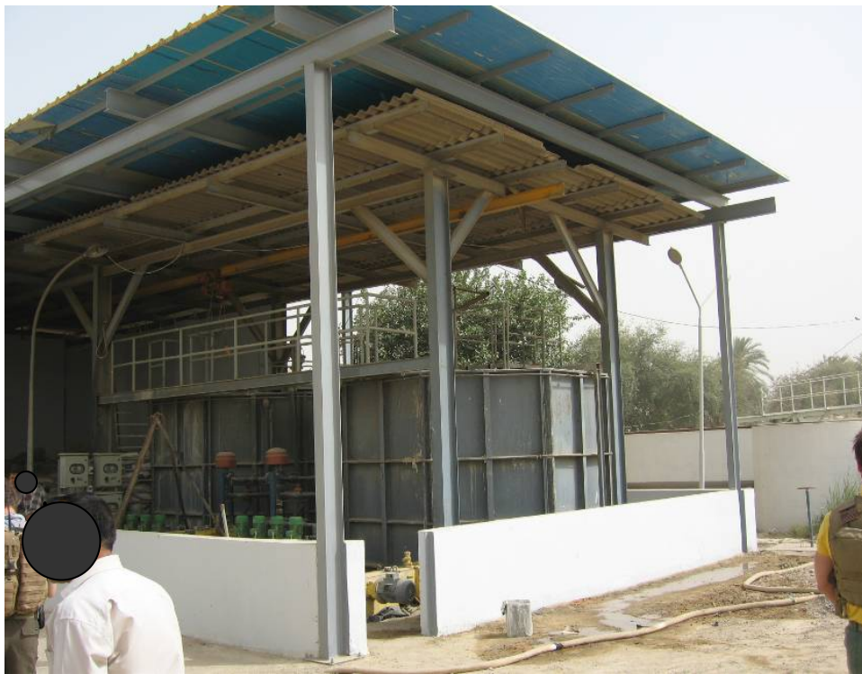
Site Photo 3: New chemical building
