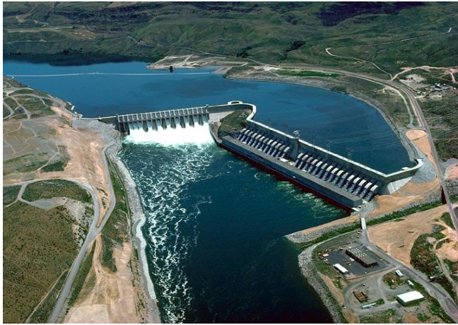
-Chief Joseph Dam on the Columbia River, WA
