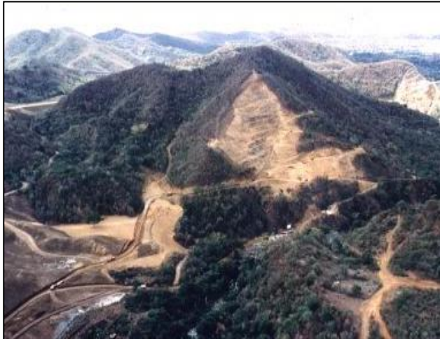
-Portugues Dam (under construction), Puerto Rico
