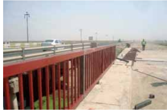
Bridge on al-Amarah–al-Maymunah Carriageway in Missan province. (USACE photo)
