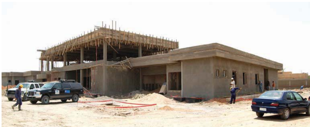
Musayib Maternity Hospital under construction in Babylon. (USACE photo)
