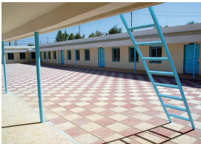
Renovated school in Erbil. (USACE photo)
