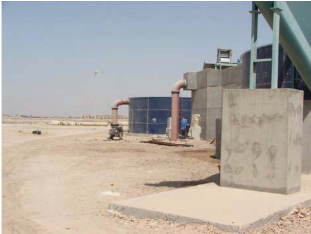
Wastewater treatment facility in Falluja.
