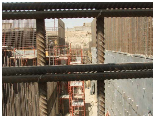
Falluja wastewater project: F1 Pump Station wall construction.
