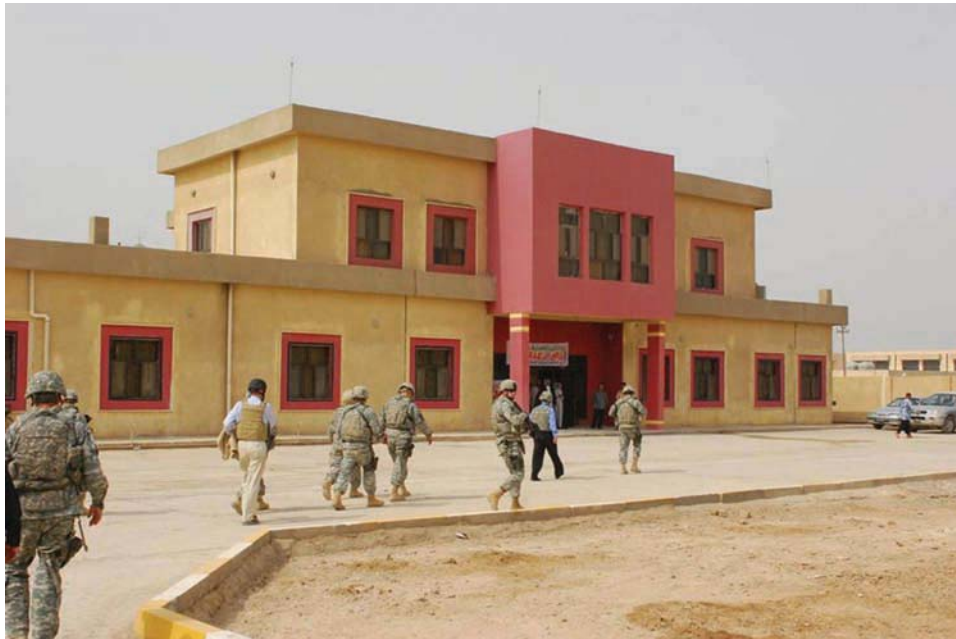
The newly completed Jamaheer clinic in Kut. (USACE photo)
