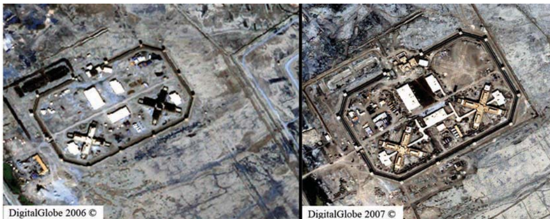
Nassriya Prison Facility. (Digital Globe 2006, 2007 photos)
