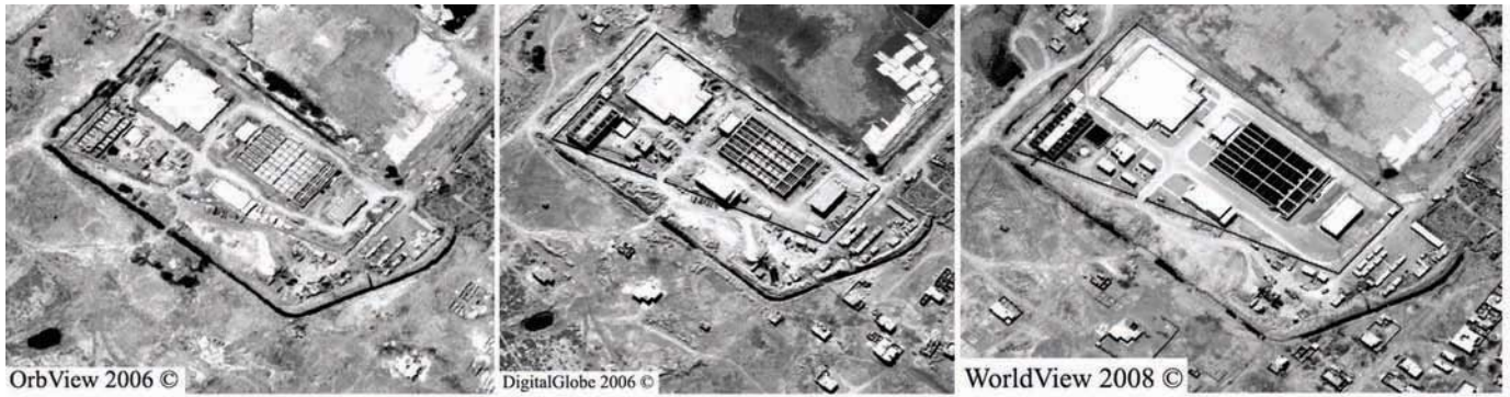
Aerial imagery of the Sadr City R3 Water Treatment Plant taken on 6/26/2006, 11/24/2006, and 5/22/2008. This quarter, SIGIR conducted an assessment of the Sadr City R3 Water Treatment Plant.
