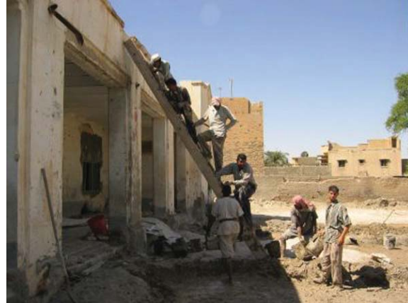
Workers repair Sajad school in Basrah. (USAID photo)
