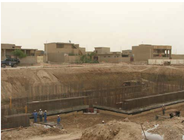
Falluja wastewater project: effluent pump station construction.
