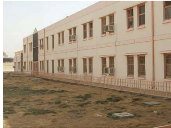
Al Faoo school: painted exterior.
