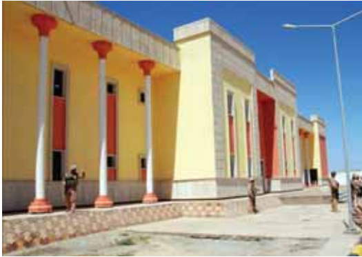
The U.S.-funded, $7.2 million al-Hillah Courthouse was designed to provide a modern complex for rule-of-law authorities in Babylon province. (USACE photo)
