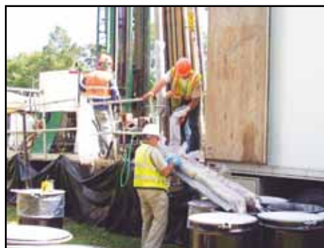
Sylvania Drill Crews Install Groundwater Profiles and Monitoring Wells
