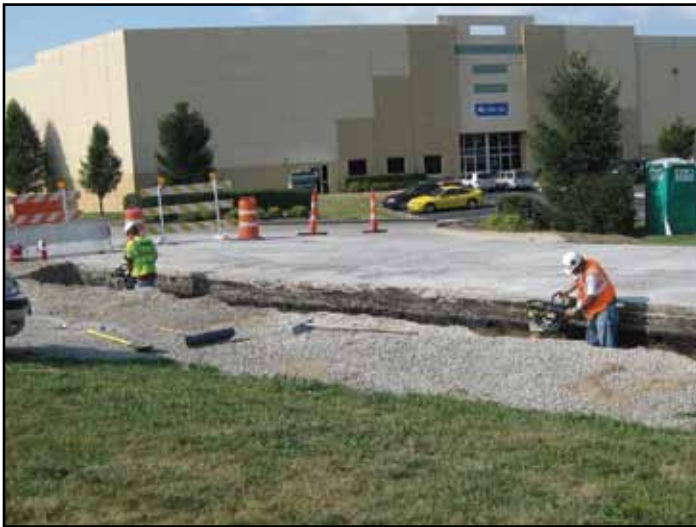
St. Louis Airport Site Vicinity Property Remediation
