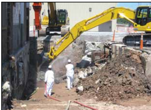
Linde Site Excavation
