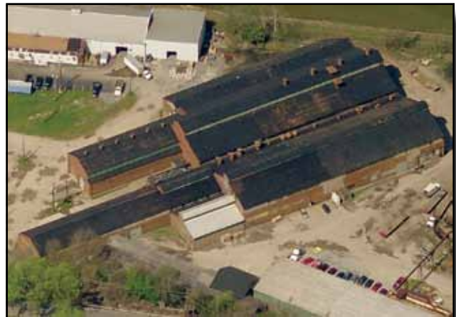
Superior Steel, Scott Township, Pa.
