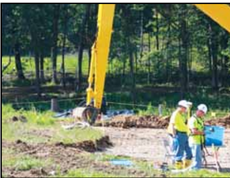
Shallow Land Disposal Area Excavation
