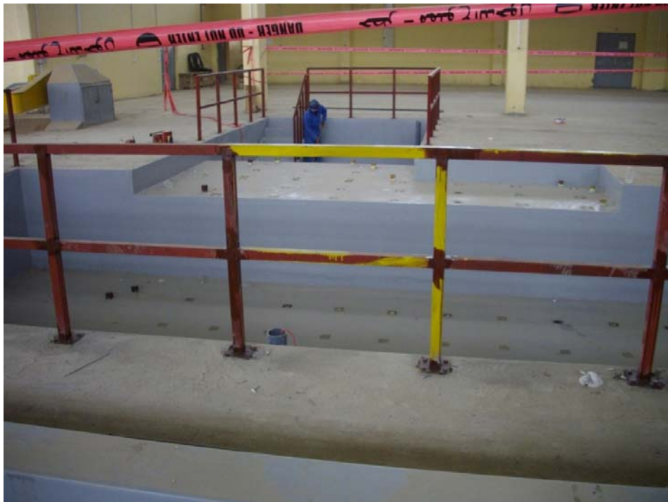
Figure 4—Photograph of Pit for Line Bore Machine
