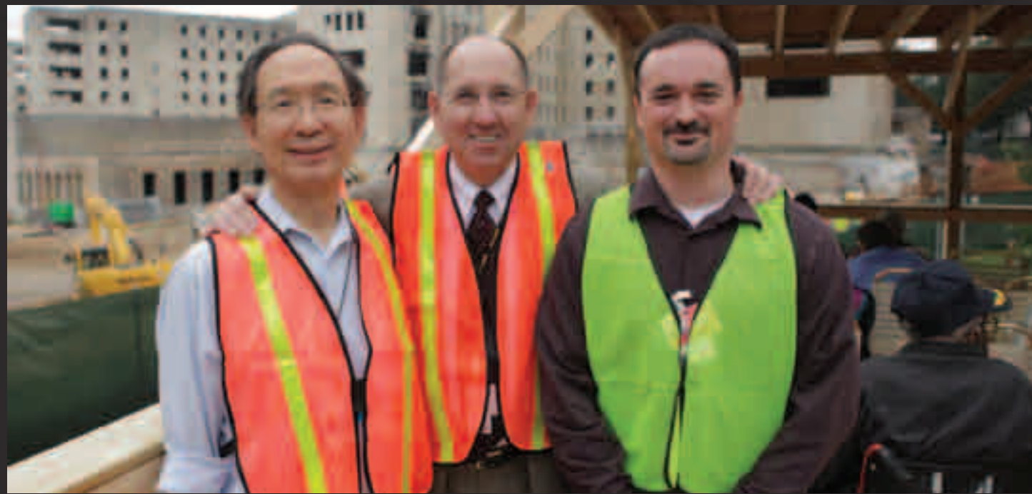
Joe Woo (Chief Architect) & Justin Seffins (Facilities Manager) join McManus at the Scott Demolition.
