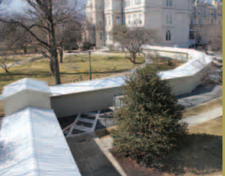
Tunnel for safe passage to interim dining hall in Sherman N. (pre-earthquake)
