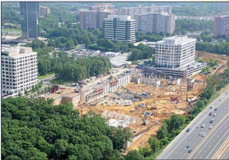
June 2009. The excavation has been completed. Pile driving has started and the first structural steel is being erected. (Photo by Marc J. Barnes)
