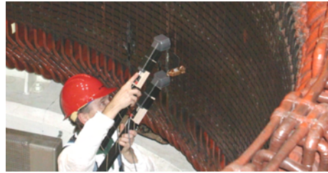
Figure 3. Generator winding insulation testing
