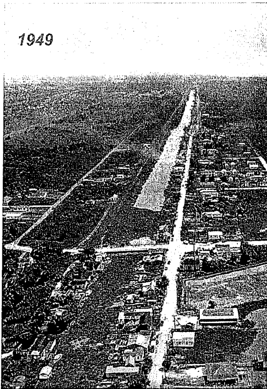
Hurricane Protection System
