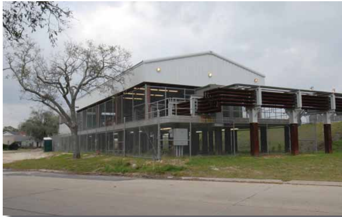
Orleans Avenue Canal - West Side - Current Condition
