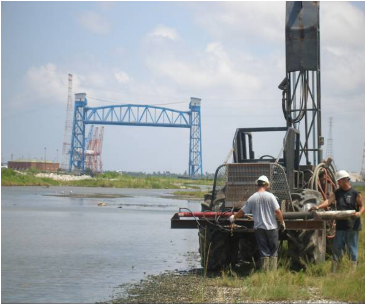
Figure 5. CME-75 Mobile Drill Rig
