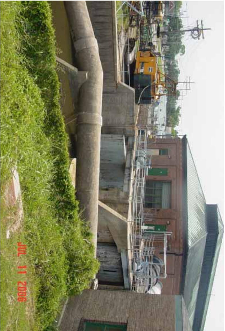
Pump Station No. 3 - Discharge into London Avenue Canal – 3000 cfs total
