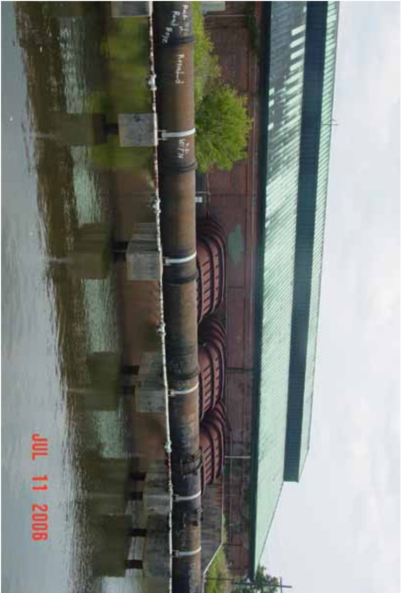
Pump Station No. 3 - Discharge into London Avenue Canal – 3000 cfs total
