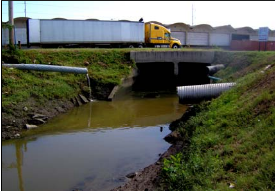
Photo No. 1 - Two 8 x 8 RCB under L&A Road
