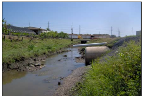
Photo No. 8 - Hoey's By-Pass Canal Discharging into Hoey's Canal
