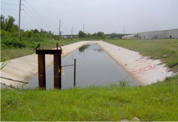
Photo No. 9 - Hoey's By-Pass Canal at L&A Road Facing Southwest
