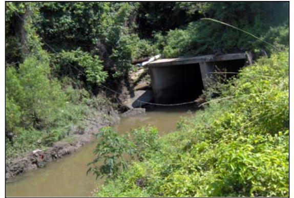
Photo No. 6 - South side of RCB Under Cold Storage Road
