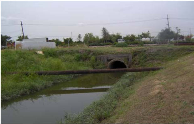
Photo No. 11 - Hoey's By-Pass entering 72" RCP under Cold Storage Rd.
