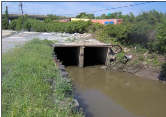
Photo No. 5 - Hoey's Canal traveling under Cold Storage Road
