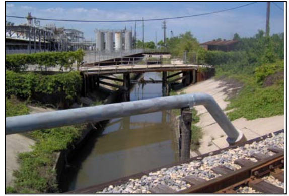
Photo No. 4 - Hoey's Canal facing Southwest at Earhart Expressway
