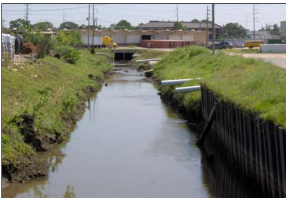
Photo No. 7 - Hoey's Canal facing Northwest toward Airline Drive
