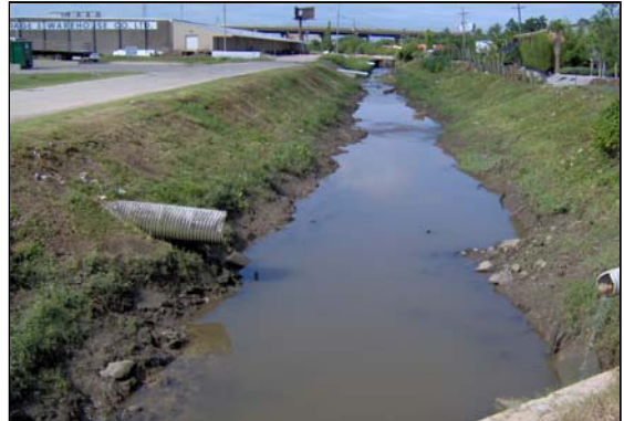
Photo No. 2 - Hoey's Canal facing Southeast from L&A Road
