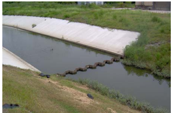
Photo No. 12 - Beginning of unlined portion of Hoey's By-Pass Canal
