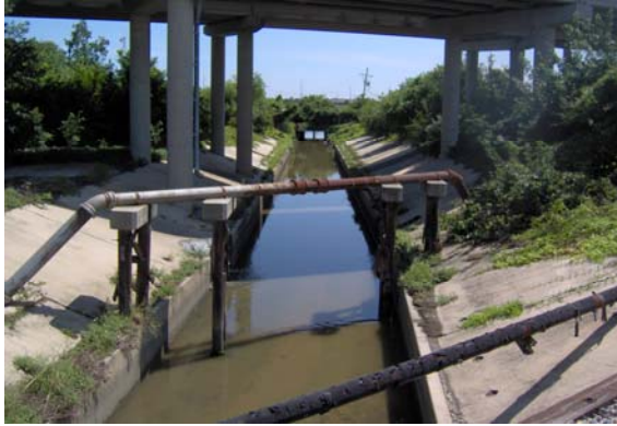
Photo No. 3 - Hoey's Canal facing Northeast at Earhart Expressway
