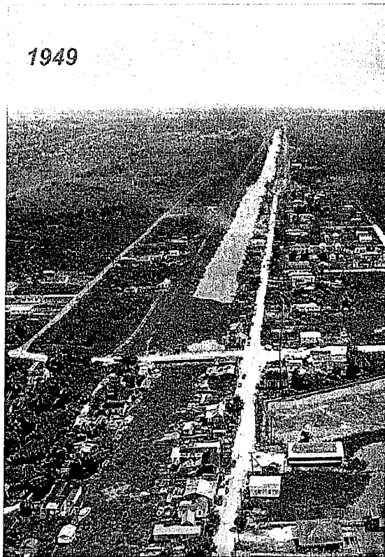
Hurricane Protection System
