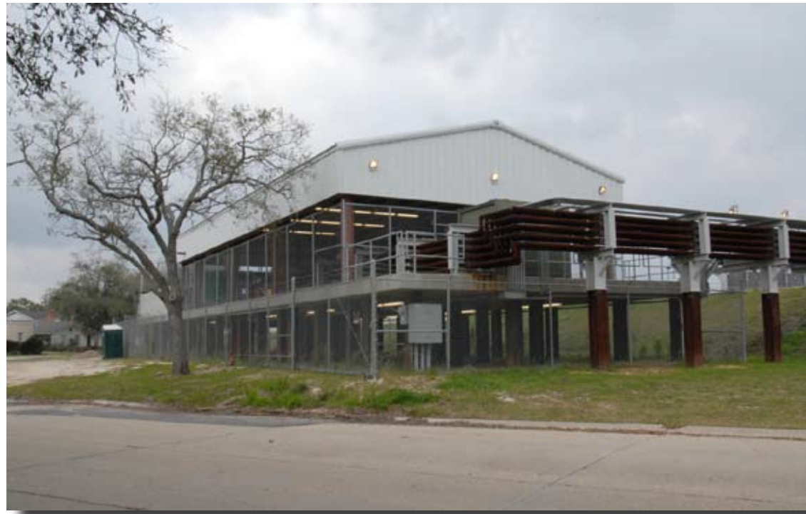
Orleans Avenue Canal - West Side - Current Condition
