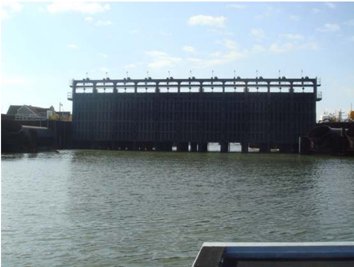
Photograph #1 17 th Street Canal Camera facing south
