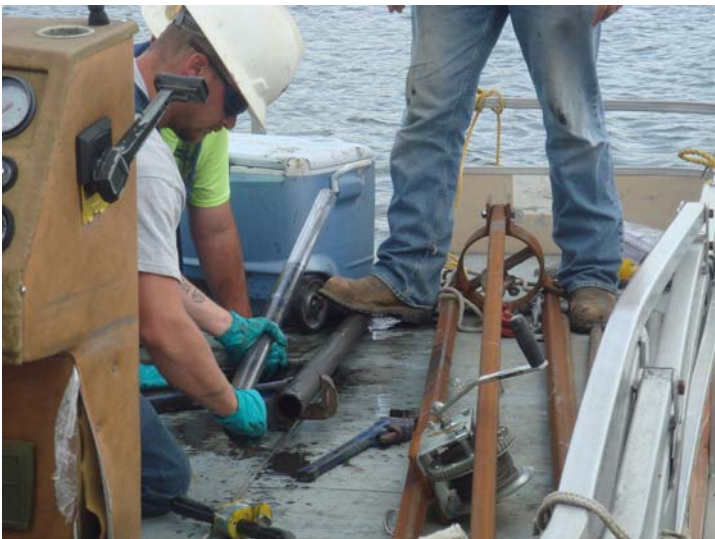
Photograph #3 Core removal at 17 th St. Camera facing east
