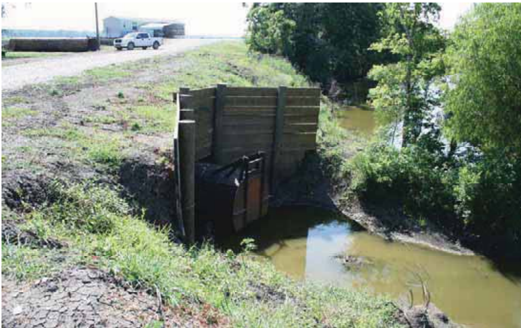
Figure 5. Discharge Flap Gate Into Bayou Tortue
