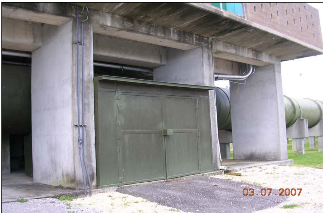
Photograph 10. Storage shed for supplies under station
