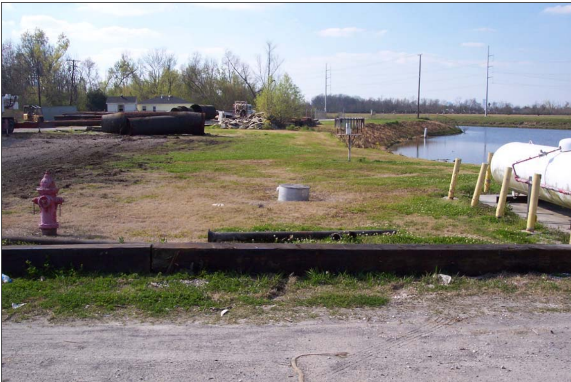
Photograph 4. Septic tank and leach field west of the pump station
