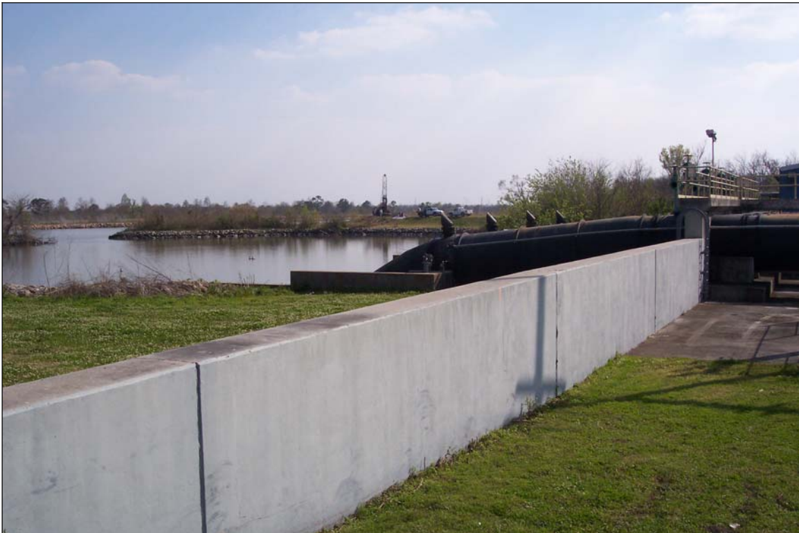
Photograph 12. View to the southeast of adjacent property
