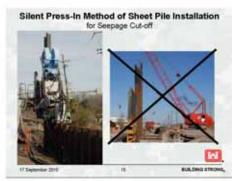
The next slide again illustrates the silent press-in method of sheet pile installation. The hydraulic machine itself is relatively silent. There is a generator that provides power for the unit, but that's a very low noise level. You won't ever see anything like this large pile driving installation like you've seen on other construction sites.
