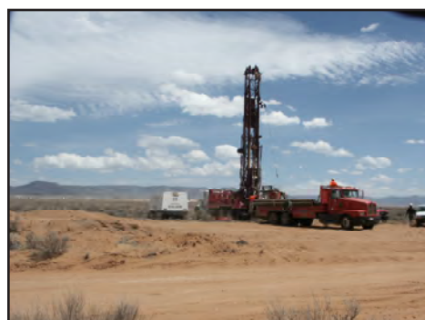
Drilling Operations at SNL/NM
