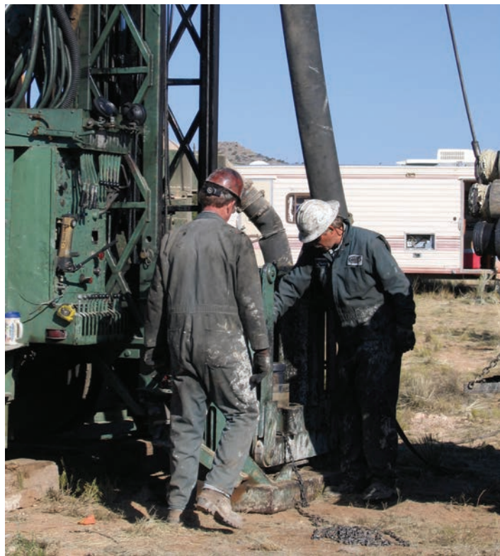
Groundwater Well Installation at SNL/NM
