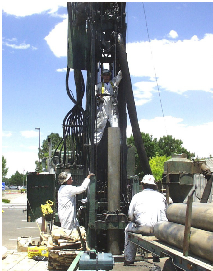
Groundwater Well Installation at SNL/NM
