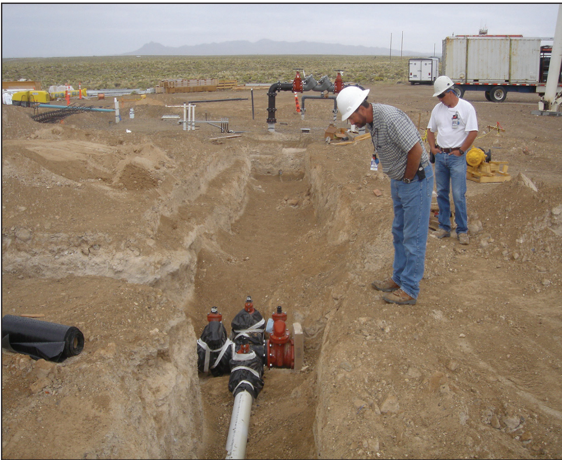
Workers inspecting the main distribution valves under the elevated water storage tower as part of the Water Distribution System Replacement Project.
