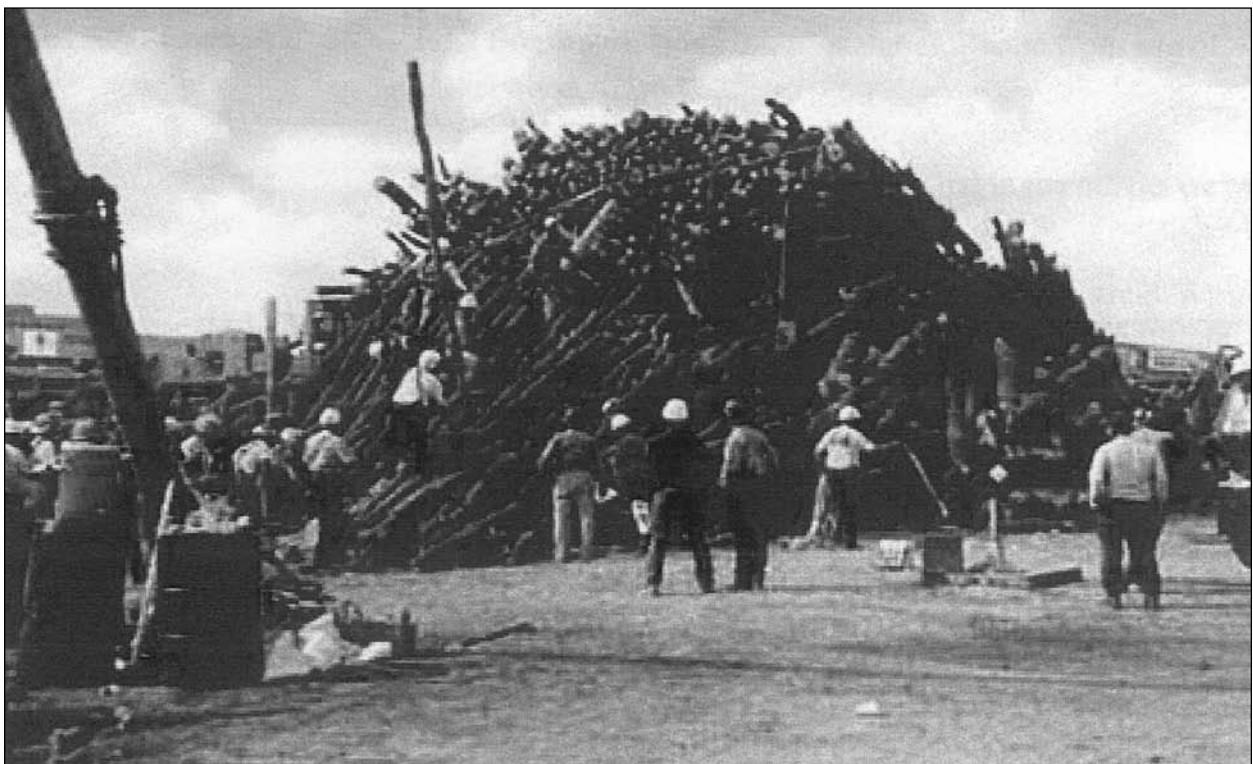
6. Day light recovery operations
