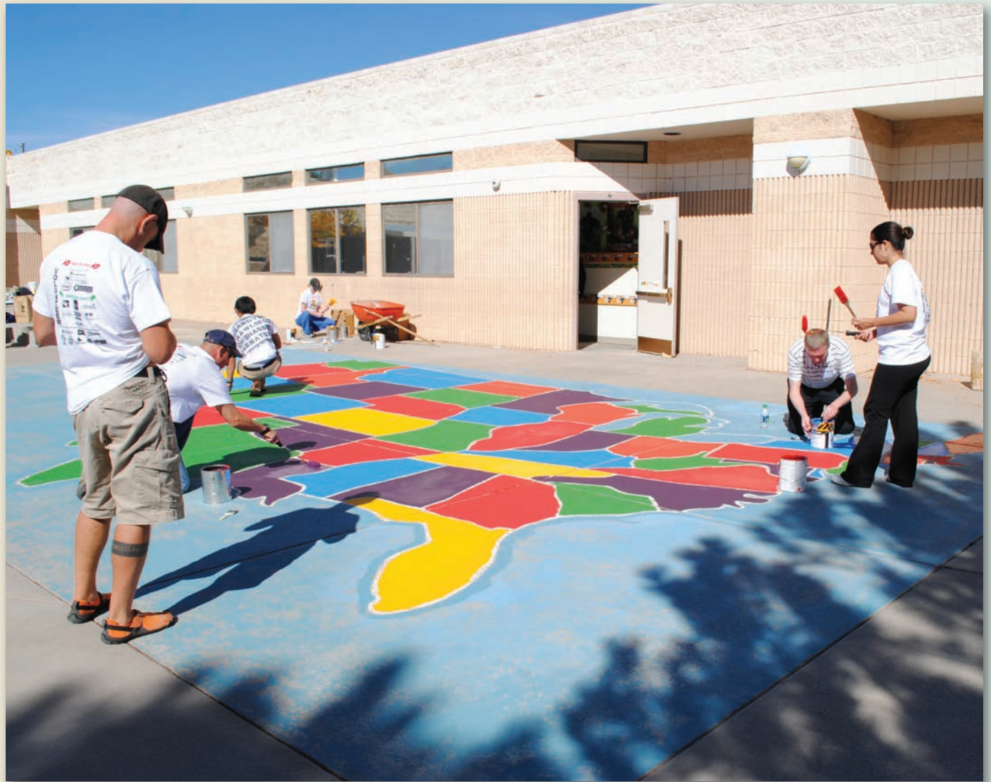
Make a Difference Day 2011 — Some 250 Sandia employees, contractors, retirees, family members, and friends volunteered to help complete projects throughout the community during Make a Difference Day. In the photo, Sandia volunteers repaint the US map on the Sandia Base Elementary School playground. (Photo by Patty Zamora)
