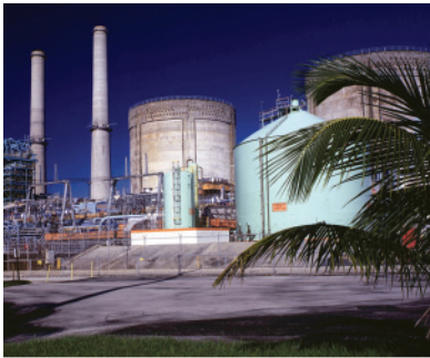
Turkey Point Nuclear Plant, Homestead, FL
