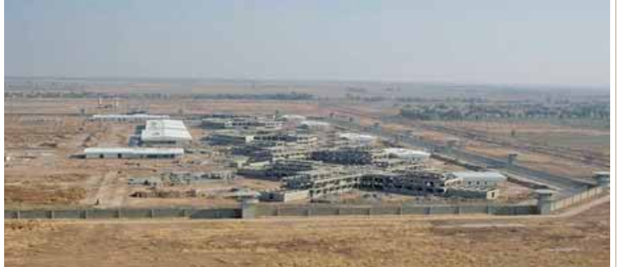
Khan Bani Sa'ad is still lying unused and incomplete. There is some discussion among local Iraqi officials that the MOJ may turn it into a working facility someday. However, as of July 2011, the MOJ has only posted a few security guards at the site, most of whom rarely report to work. (USACE photo)
