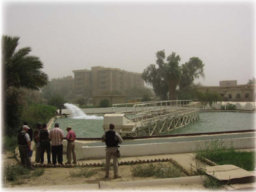
TREATMENT FACILITY INSPECTION – An engineer and auditor from a Special Inspector General for Iraq Reconstruction (SIGIR) assessment team inspect a settling tank at a central Iraq water treatment plant.
