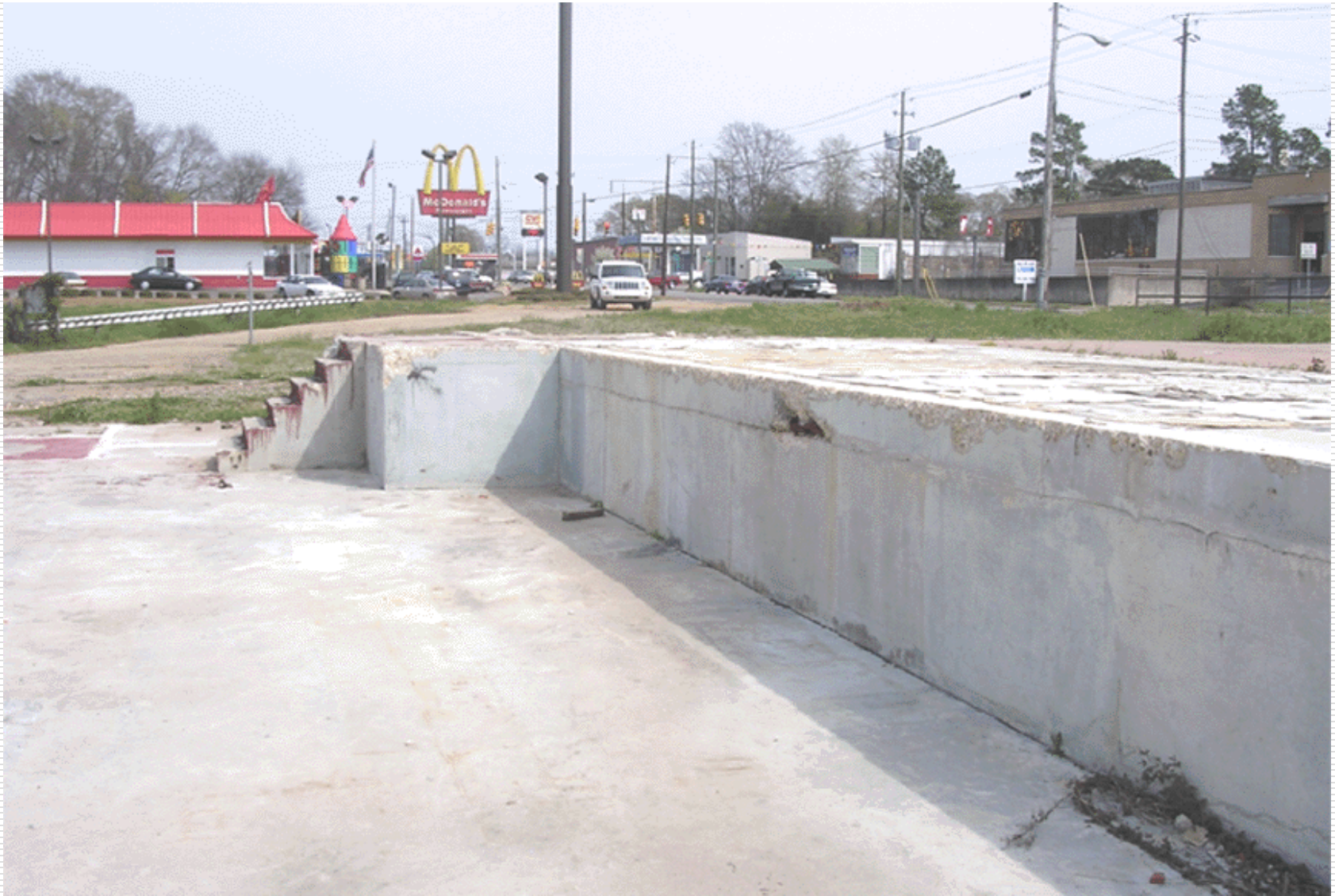
genetta park site former conditions: after existing structure's demolition
