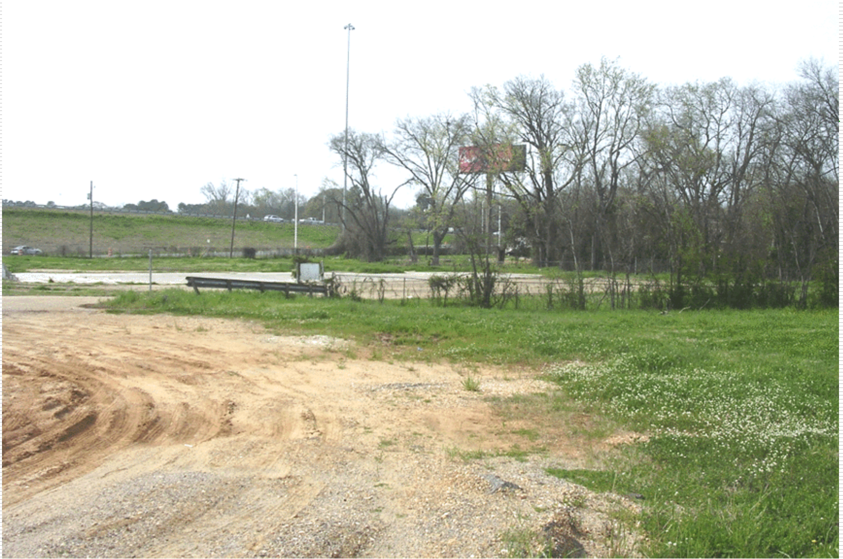
genetta park site current conditions: foundation removed, site graded & vegetated
