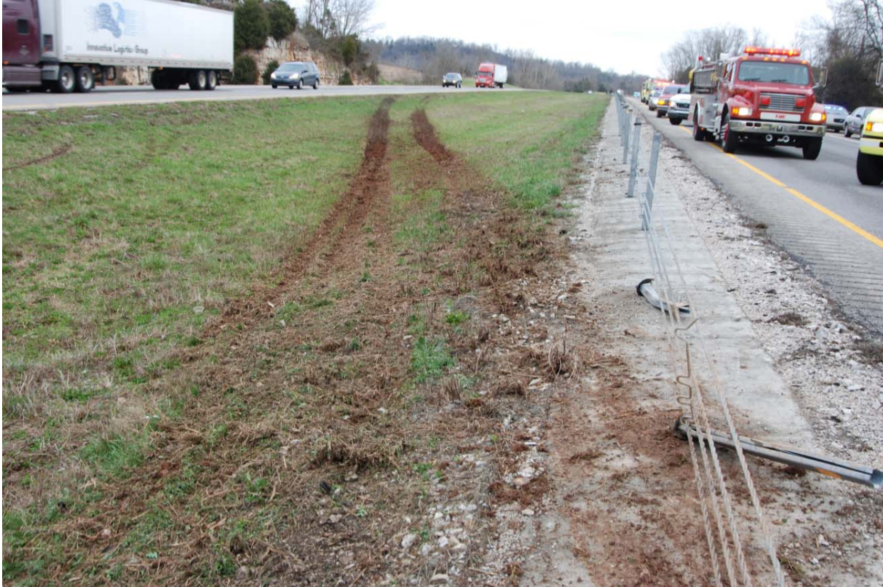
Figure 3. Truck's oncoming crossover path, viewed from the edge of the northbound passing lane.
