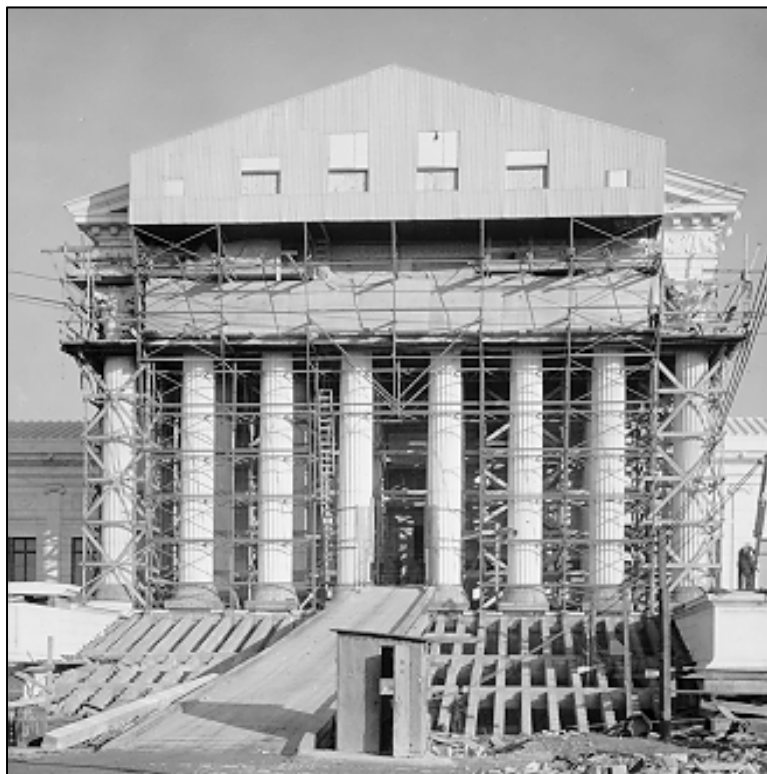
The West Pediment under construction – January 4, 1934 Photograph by Commercial Photo Company
