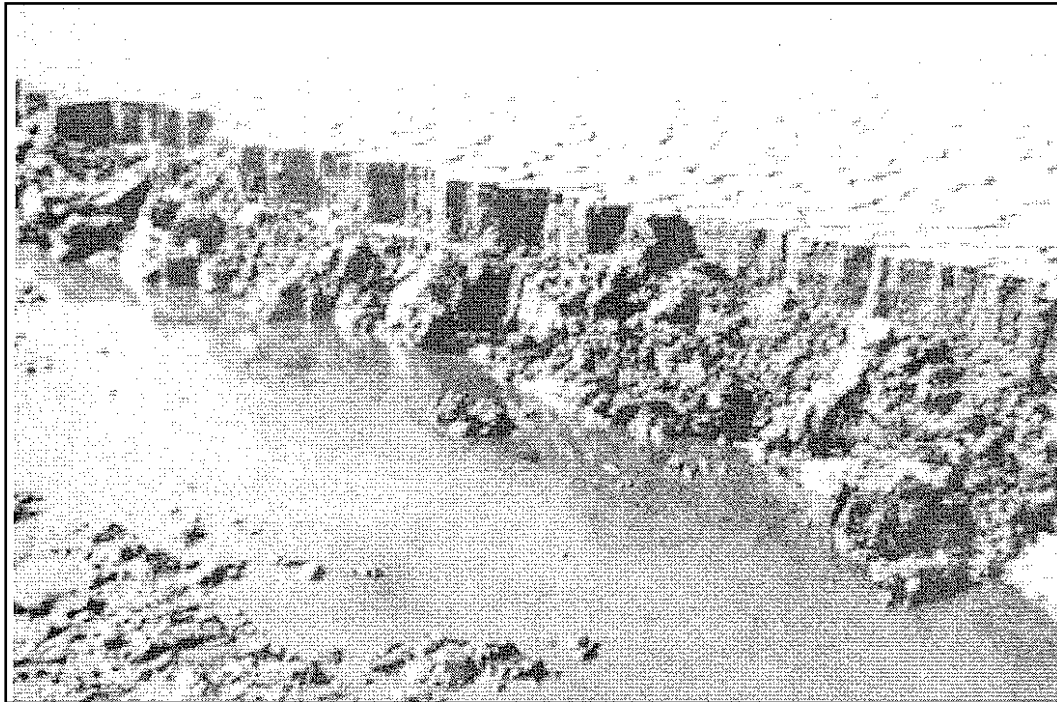
Figure B7. Desiccation crust adjacent to perimeter 3- to 5-foot-deep drainage trench.
