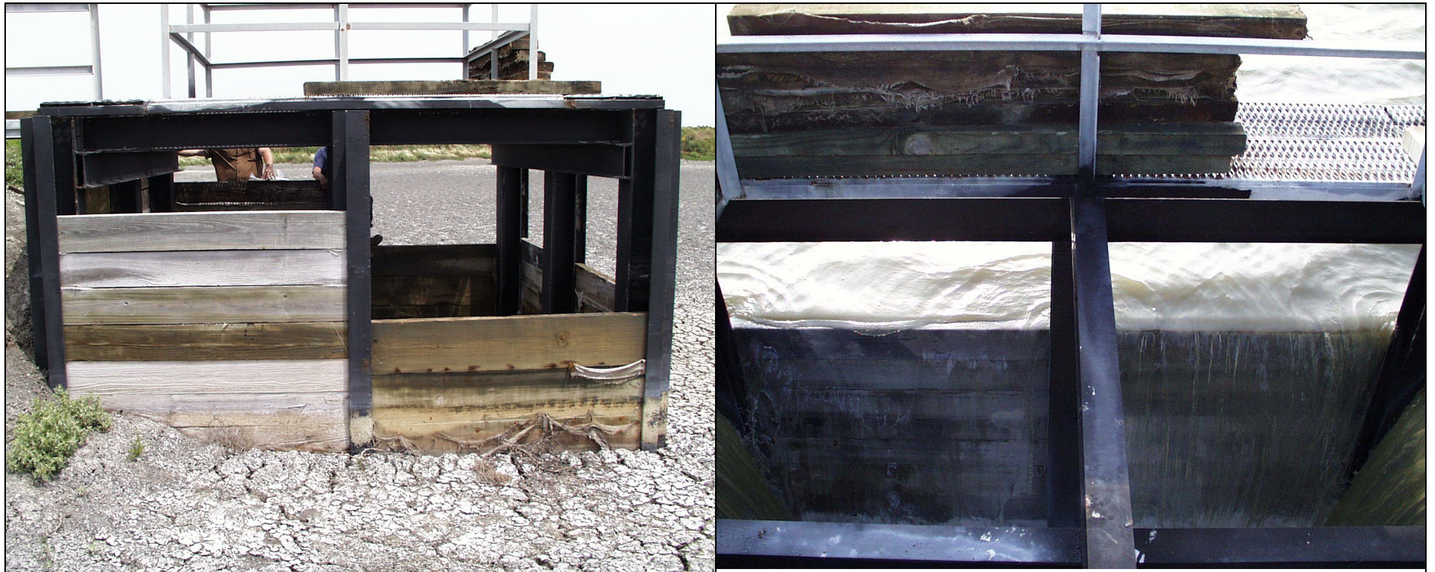
Figure 26. Box weir structure.
