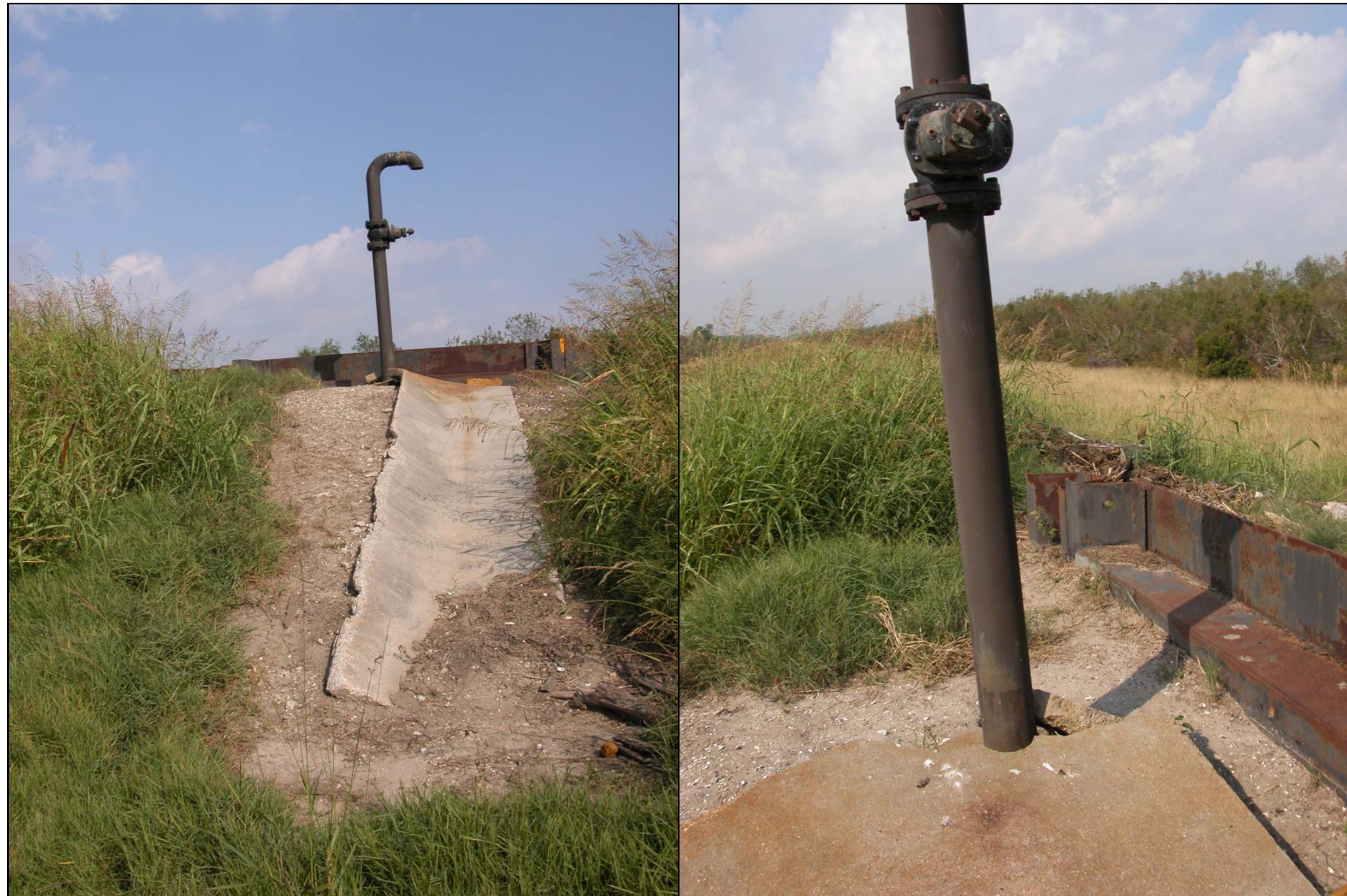
Figure 25. Pipeline Protection Structures.
