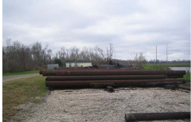
Photograph 8. Example of a proposed safe room location in a highly disturbed area at Planters Pump Station (photograph taken on February 2, 2007).
