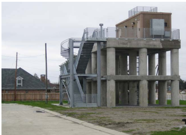
Photograph 2. Completed safe room constructed at the Bonnabel Pump Station (photograph taken on February 2, 2007).
