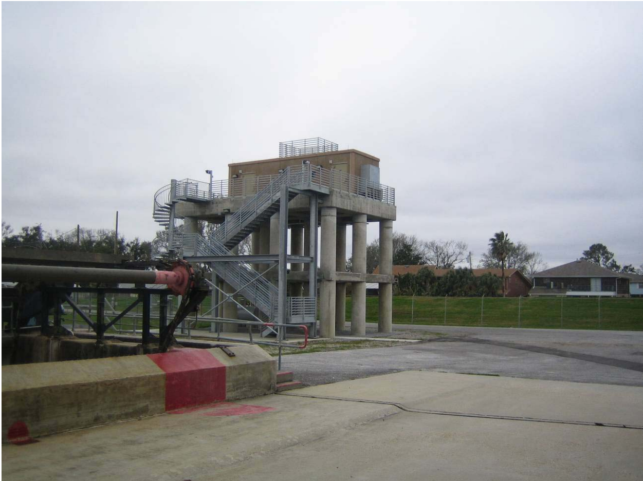
Safe room located at the Bonnabel Pump Station in Jefferson Parish, Louisiana (photograph taken on February 2, 2007).
