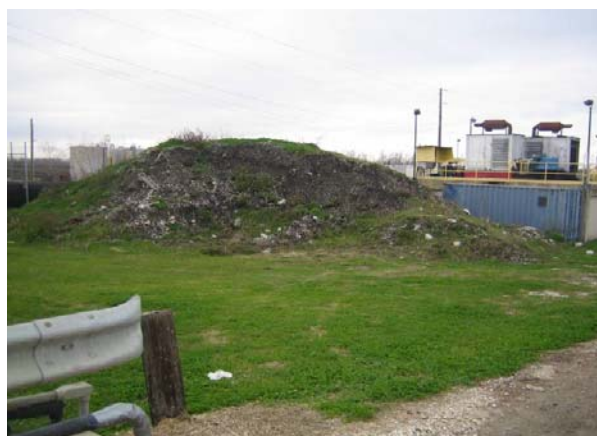
Photograph 6. Location of proposed safe room at Lake Cataouatche Pump Station (photograph taken on February 2, 2007).
