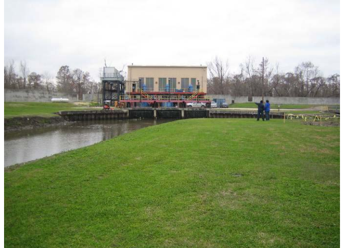
Photograph 7. Example of a proposed safe room location along a canal bank at Westwego #2 Pump Station (photograph taken on February 2, 2007).
