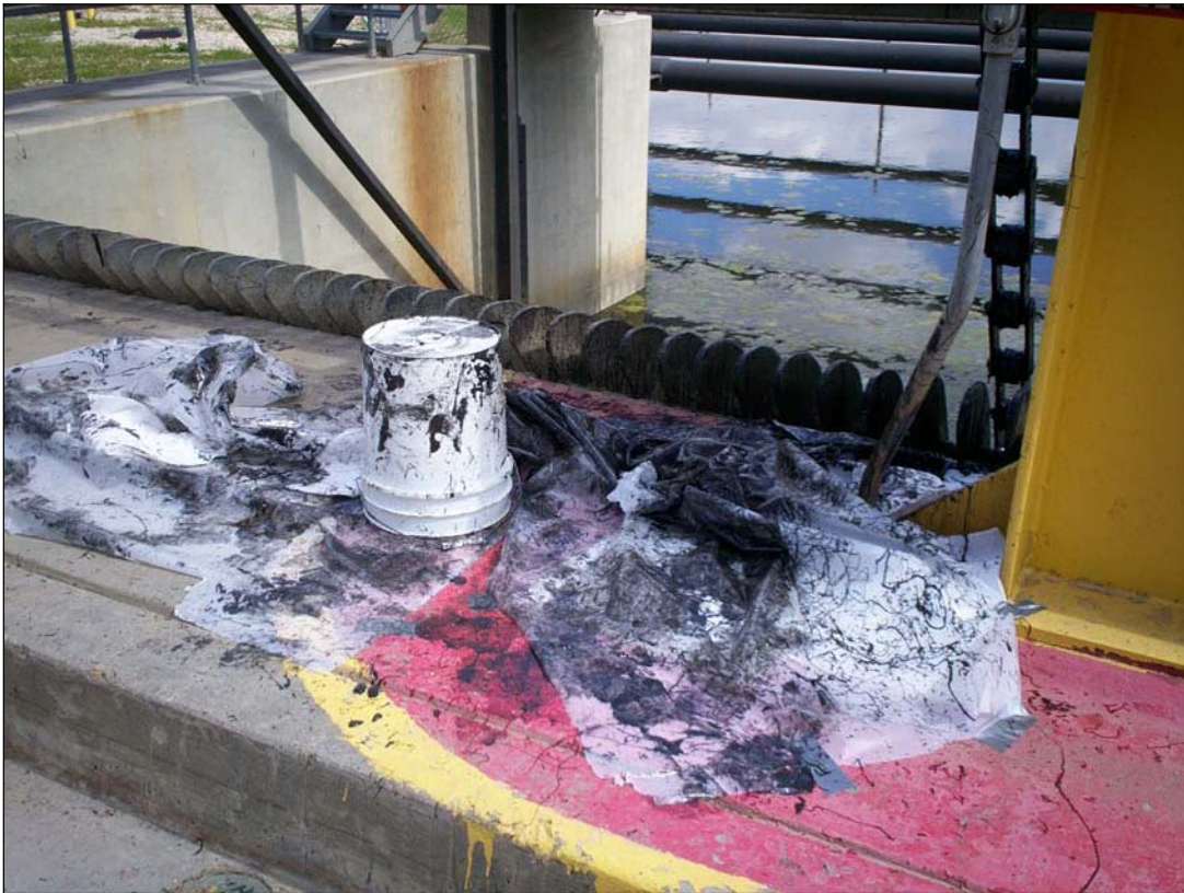
Photograph 3. Lubricating gear grease spill adjacent to debris screen
