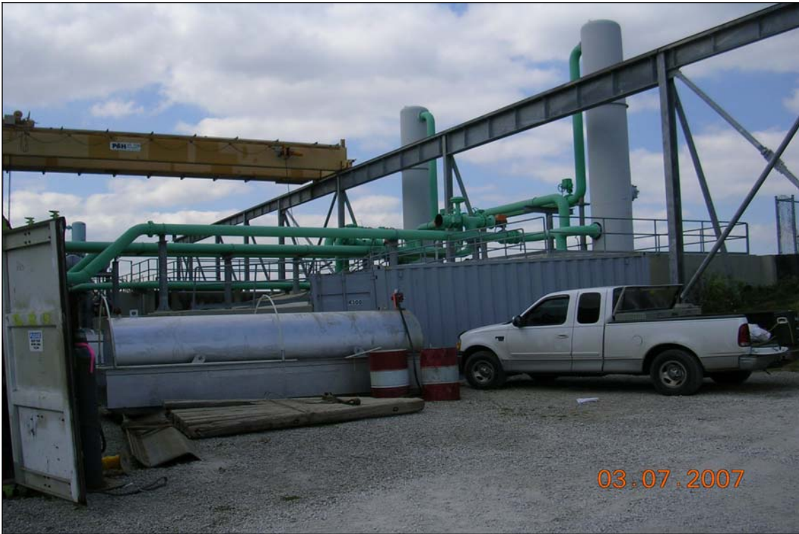
Photograph 3. Fuel tank in containment basin for levee repair equipment
