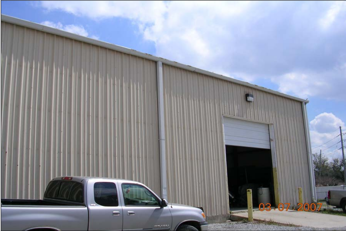
Photograph 1. Warehouse and office structure on subject property
