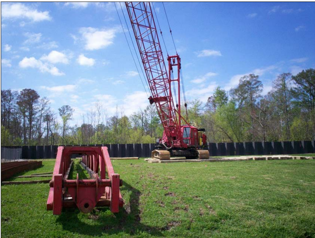
Photograph 6. Construction equipment on subject property
