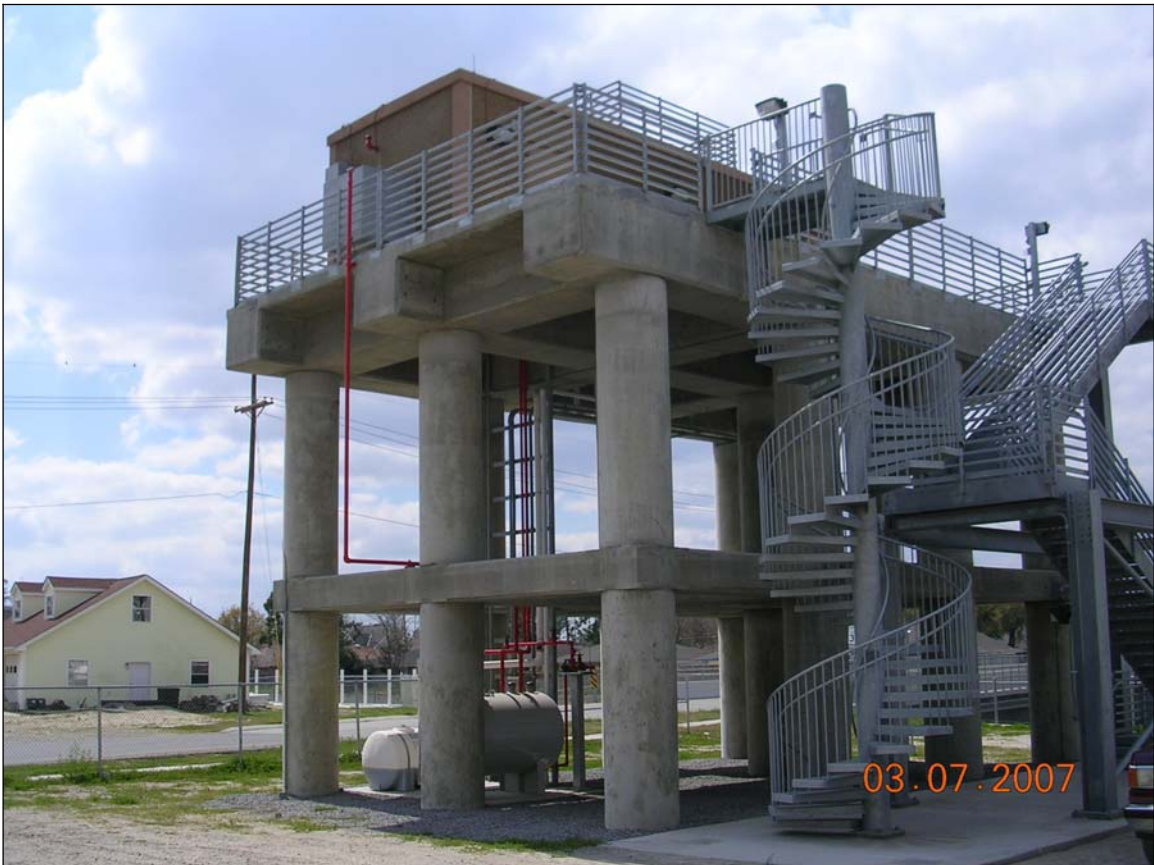
Photograph 2. Safe room and diesel storage tanks underneath
