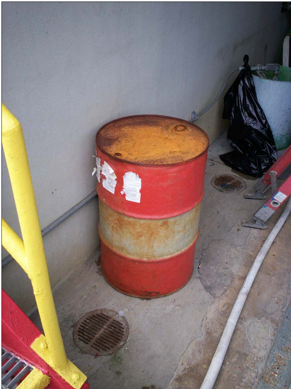
Photograph 16. Oil drum inside pump station
