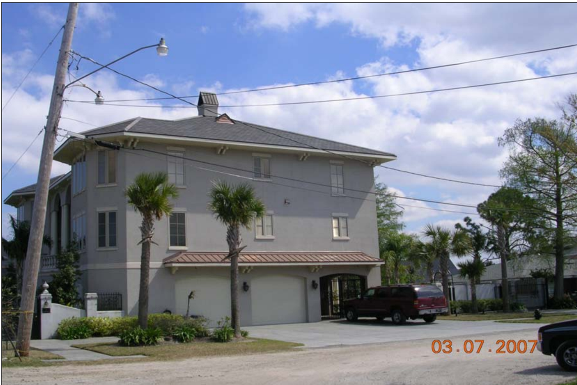
Photograph 10. View of adjacent property to the east
