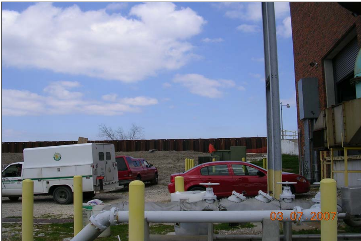
Photograph 5. Historic LUST site on subject property
