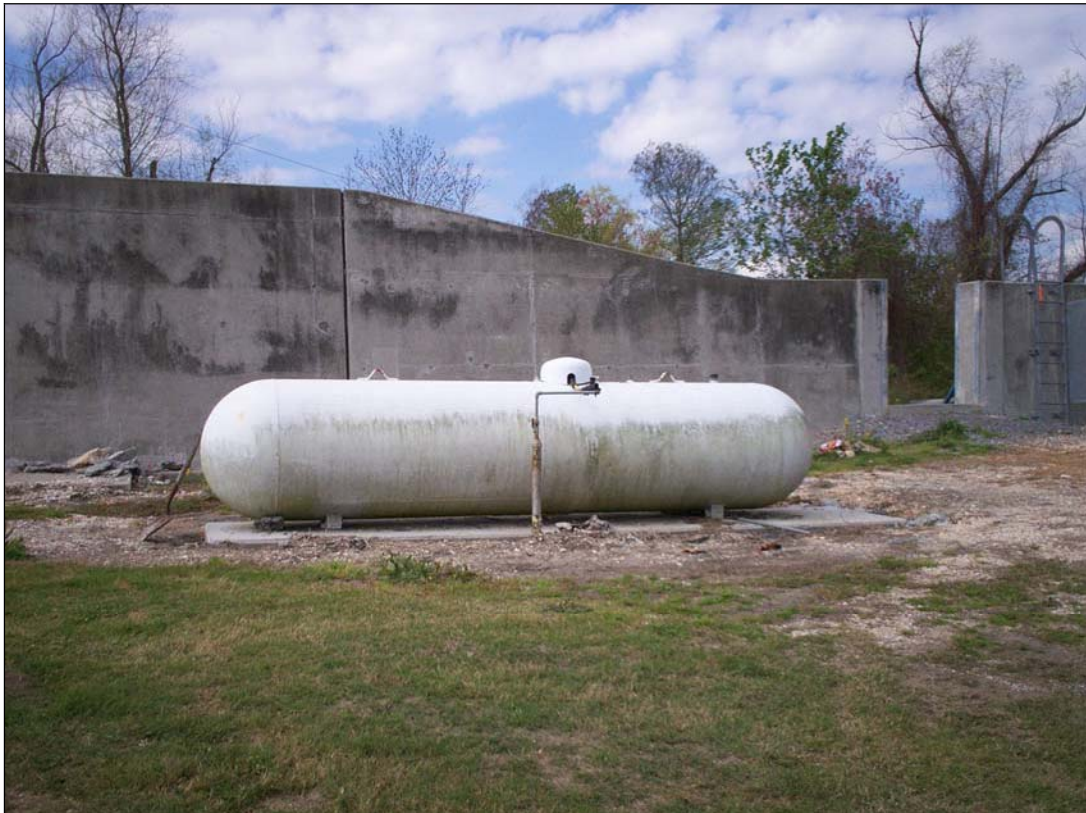
Photograph 2. Propane tank on subject property
