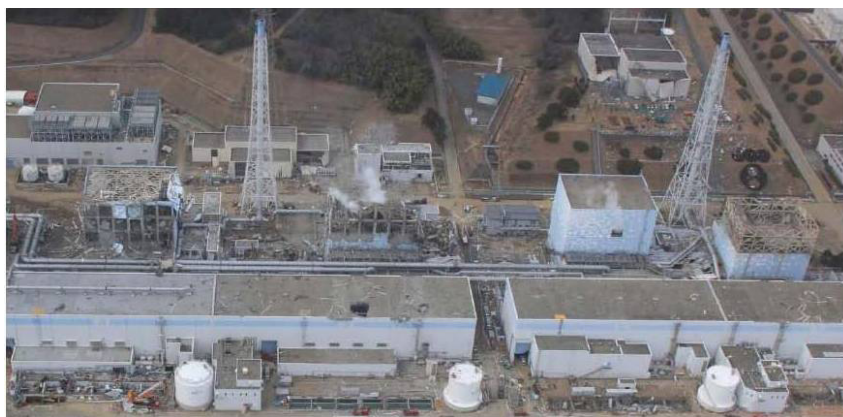
Figure 7: Fukushima Dai-ichi Units 1–4 following explosions
