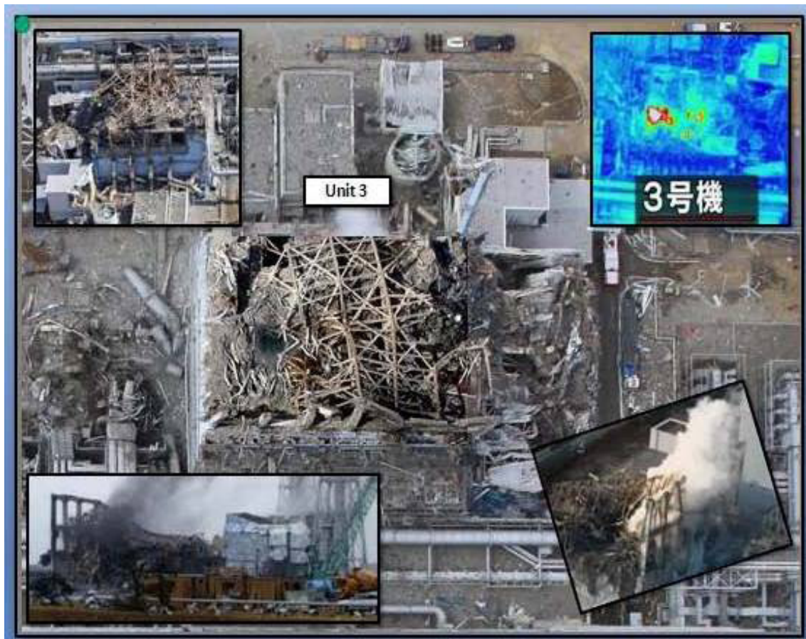
Figure 5: Damage to Unit 3
