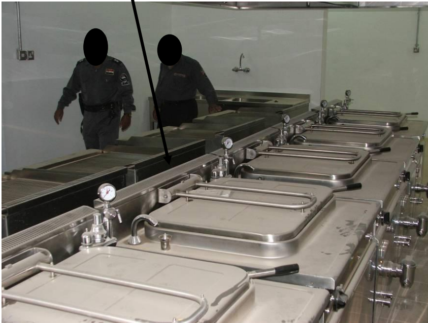
Site Photo 18. Ovens and grills within the kitchen area
