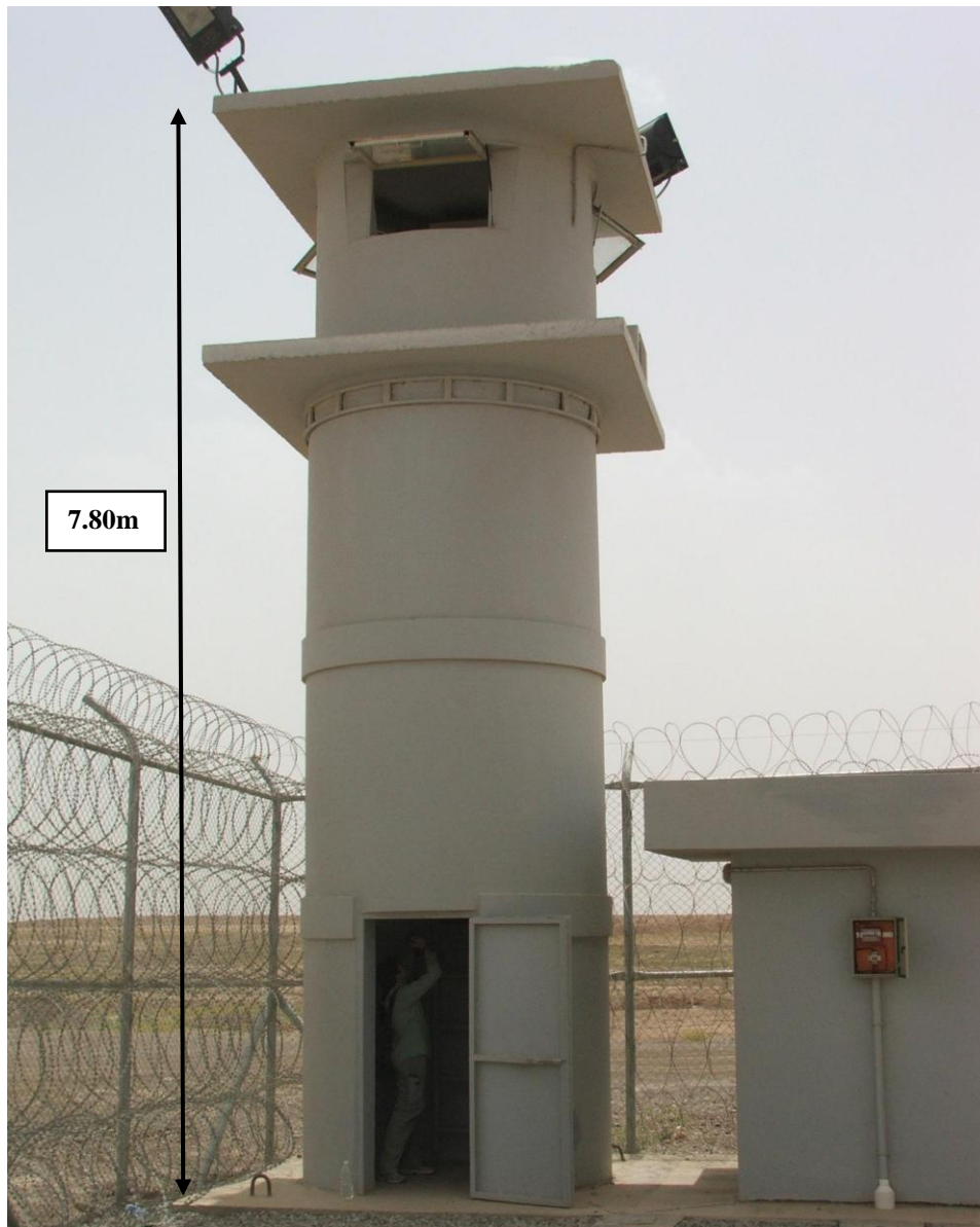
Site Photo 7. Guard tower, which provides 360-degree coverage of surrounding areas
