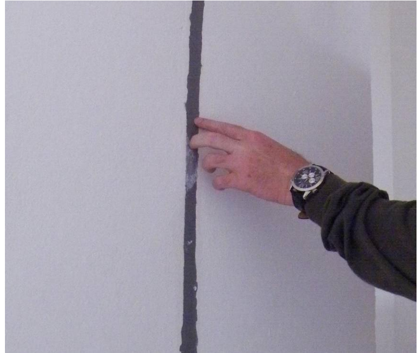
Site Photo 24. SIGIR checking quality of expansion joint material
