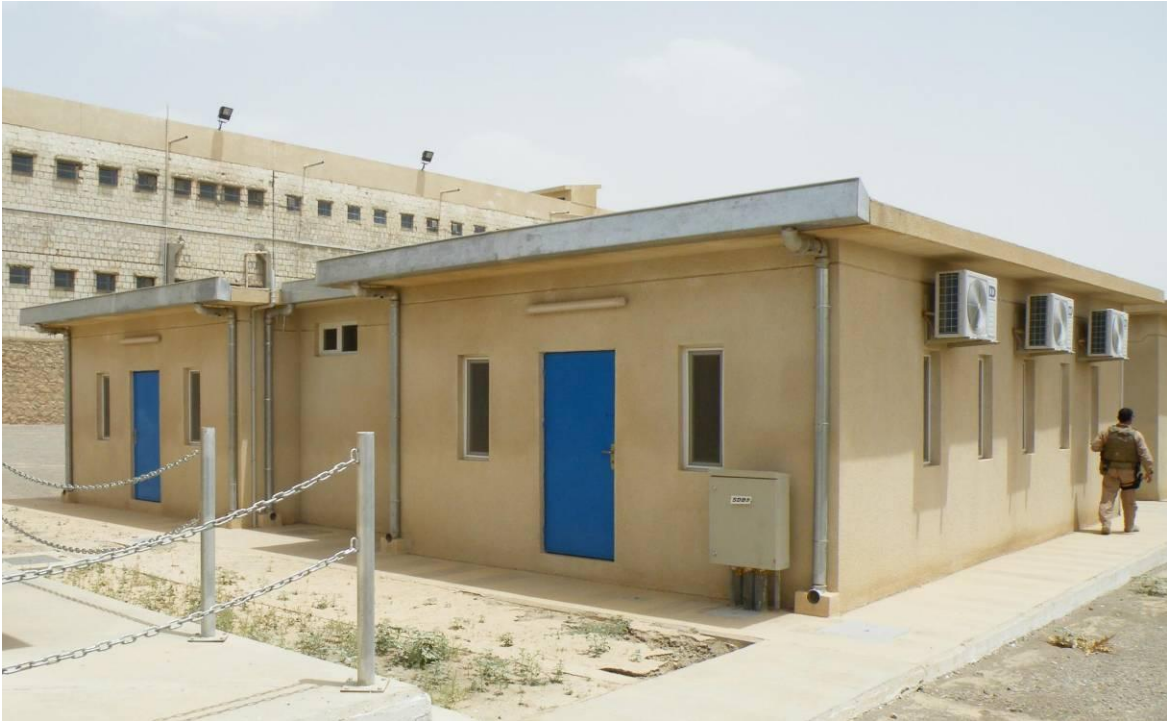
Site Photo 8. Exterior view of guard barracks building
