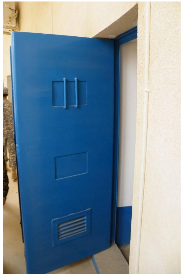
Site Photo 16. Steel prison cell door
