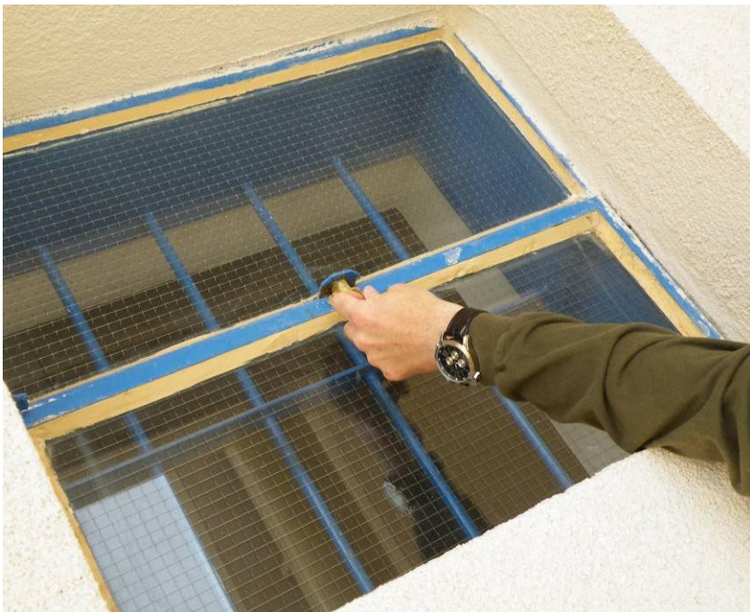
Site Photo 15. Security features for prisoner cell windows
