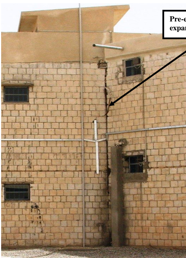
Site Photos 25 and 26. Pre-existing external expansion joints
