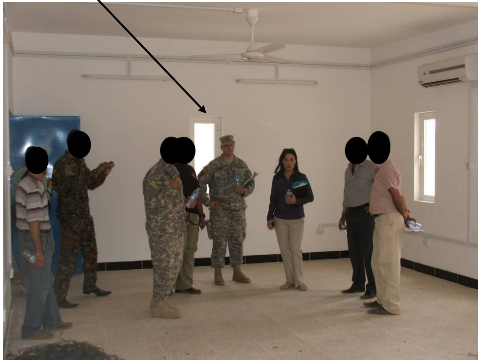
Site Photo 9. Interior view of the Type B guard barracks building room
