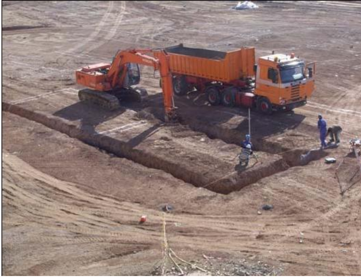
Site Photo 3. Excavation of guard barracks building (Courtesy of USACE)
