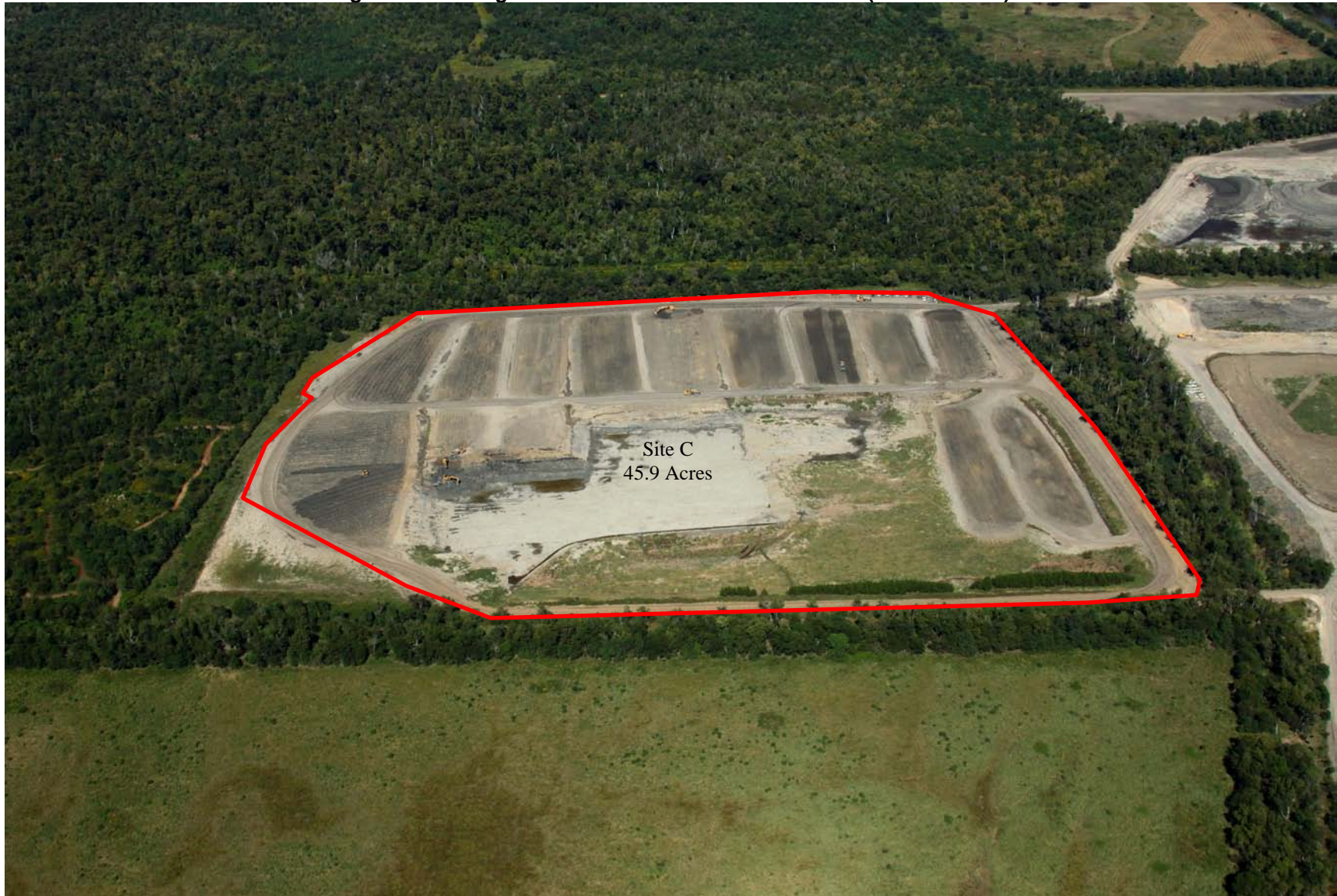
Figure 6. Existing Conditions for Stabilized Soil Site C (October 2010)
