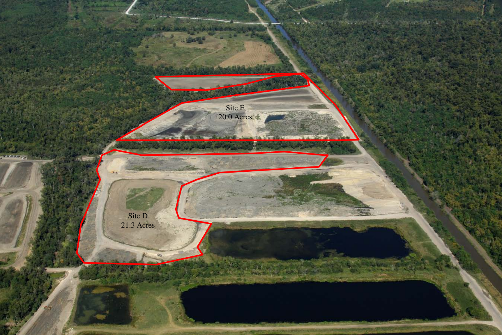
Figure 7. Existing Conditions for Stabilized Soil Mixing Sites D and E (October 2010)
