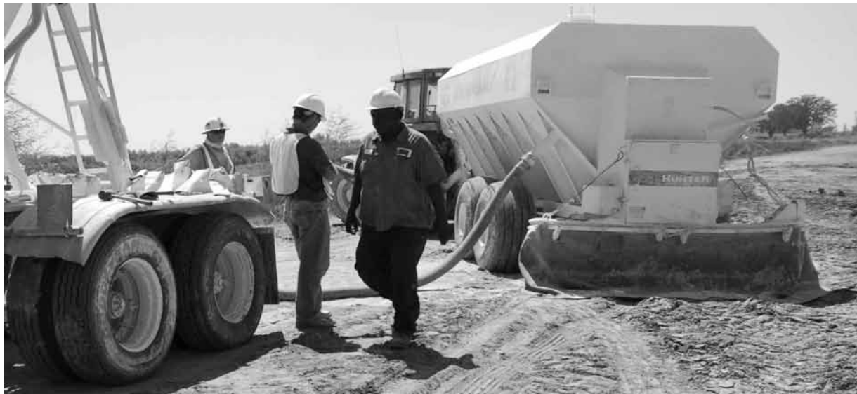
Figure 14. Material Loading onto Spreader
