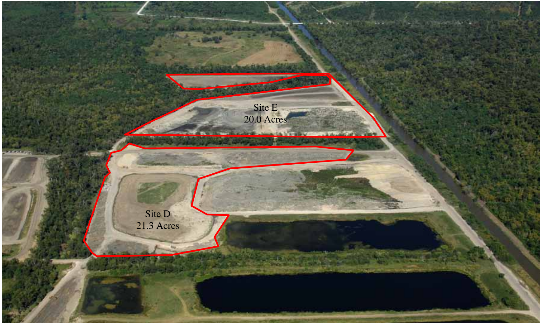
Figure 12. Aerial View of Sites D and E at Walker Road Soil Mixing Area
