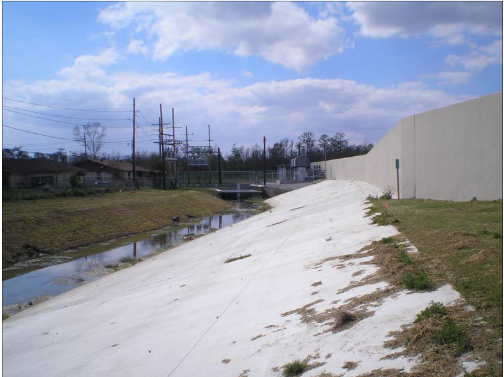
Photograph 20. View of Mt. Kennedy pump station to the southwest
