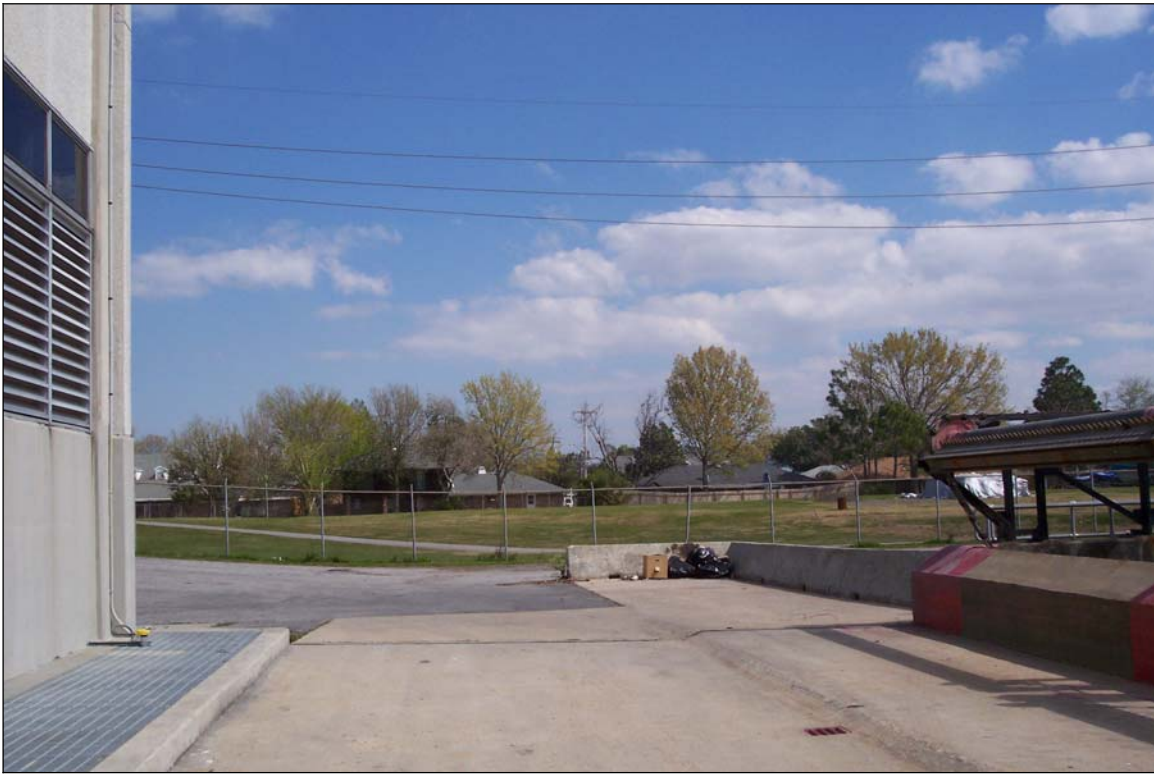
Photograph 5. View of adjacent property to the east
