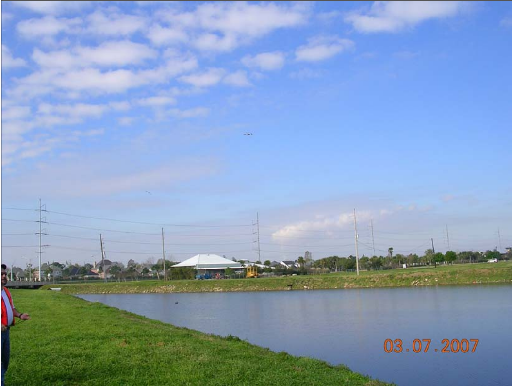
Photograph 9. Intake basin south of pump station
