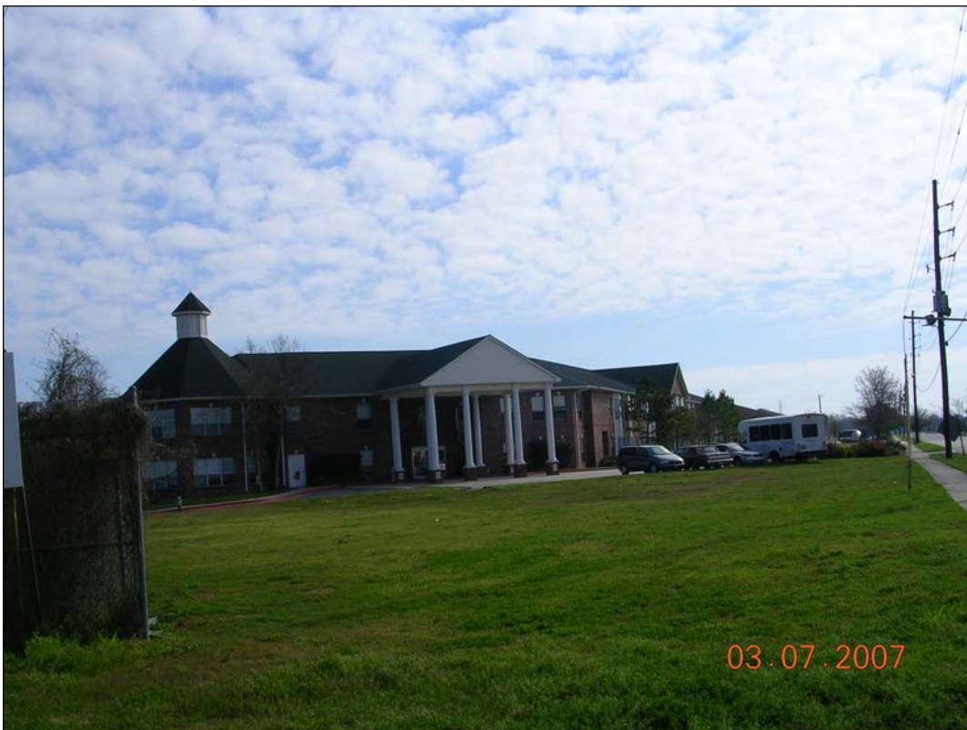
Photograph 10. View of adjacent property to the east
