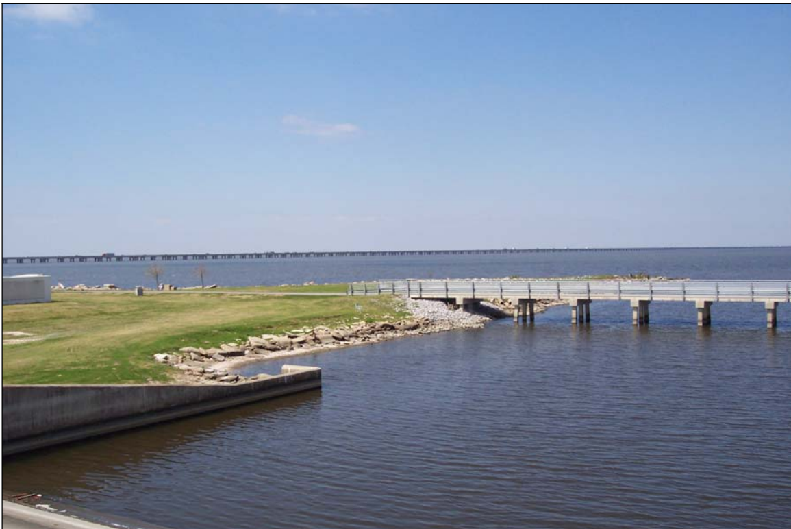
Photograph 8. View to the northwest from outfall basin
