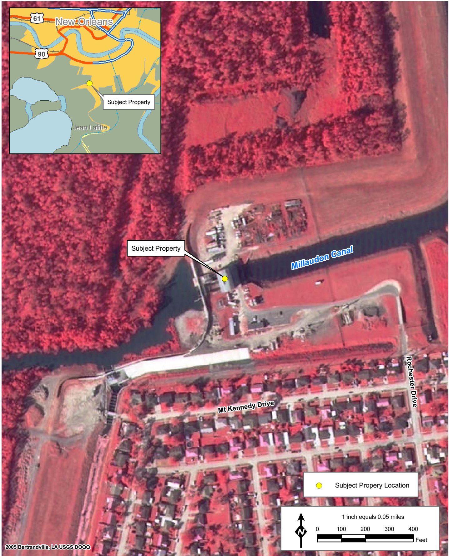
Figure 3: Ames Pump Station Area
