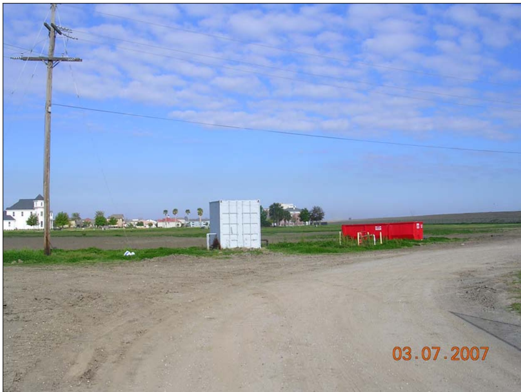
Photograph 6. Well pump house on subject property
