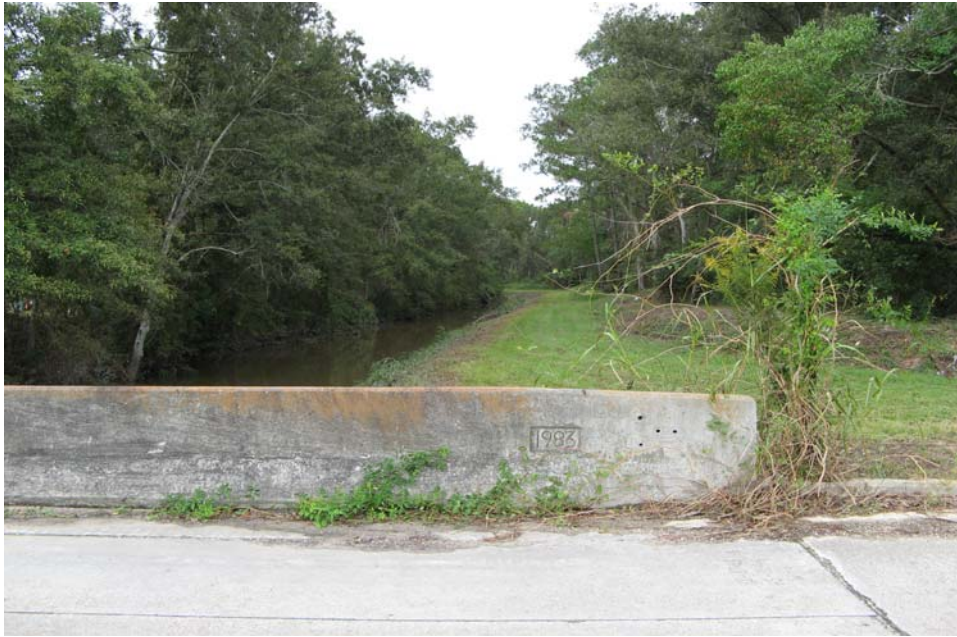
Figure 3. Photo of the W-14 Canal, looking north from the Daney Street Bridge. Proposed Daney Street detention pond is on the right side of the photo.
