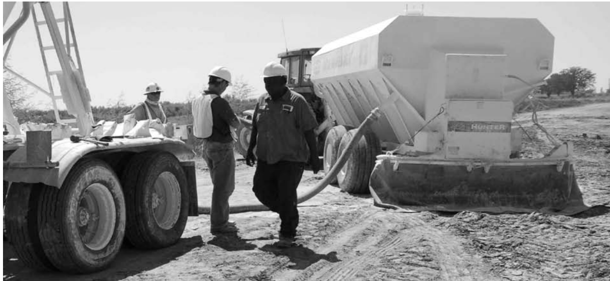
Figure 14. Material Loading onto Spreader
