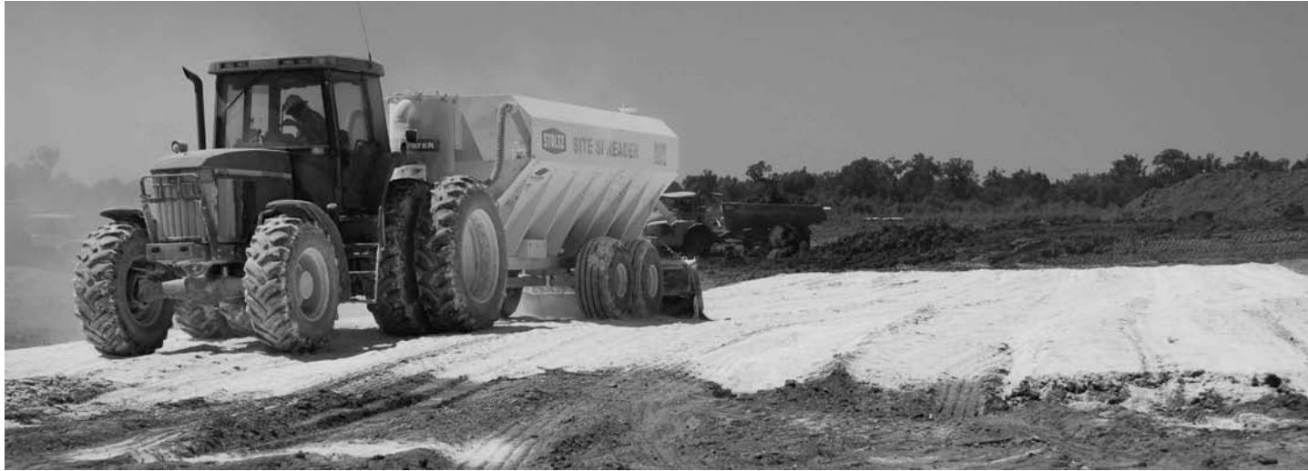
Figure 15. Lime Spreader Depositing Material
