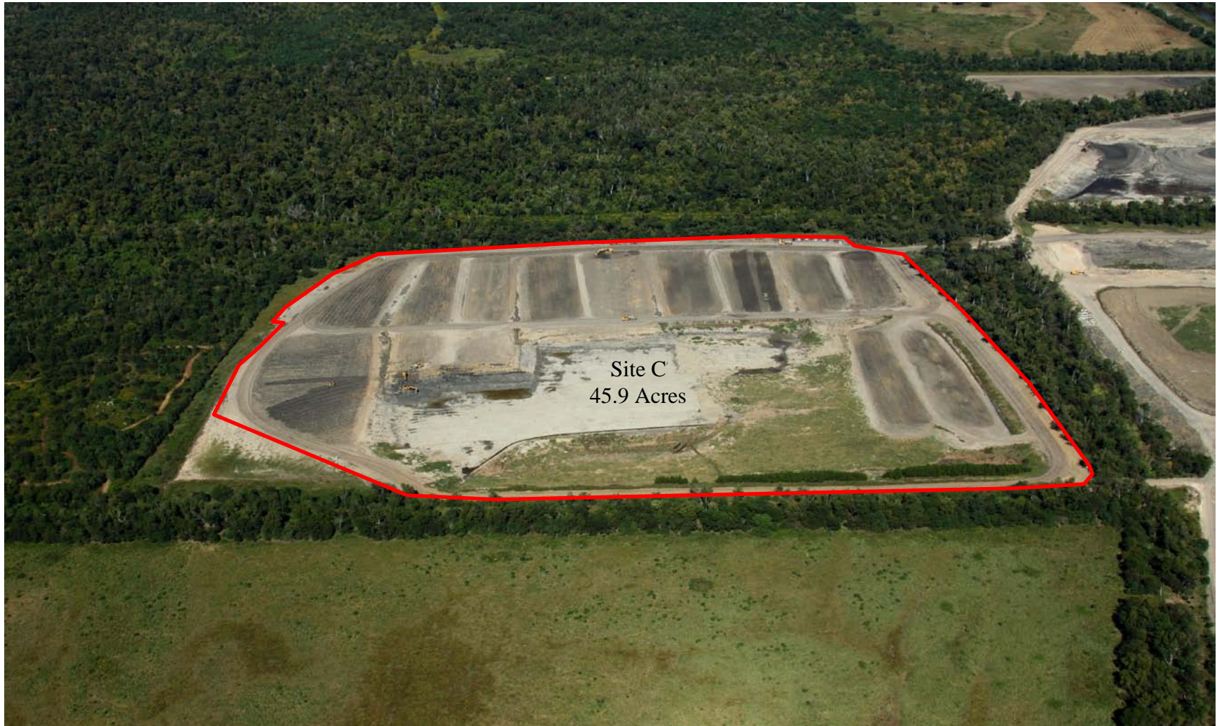
Figure 11. Aerial View of Site C at Walker Road Soil Mixing Area
