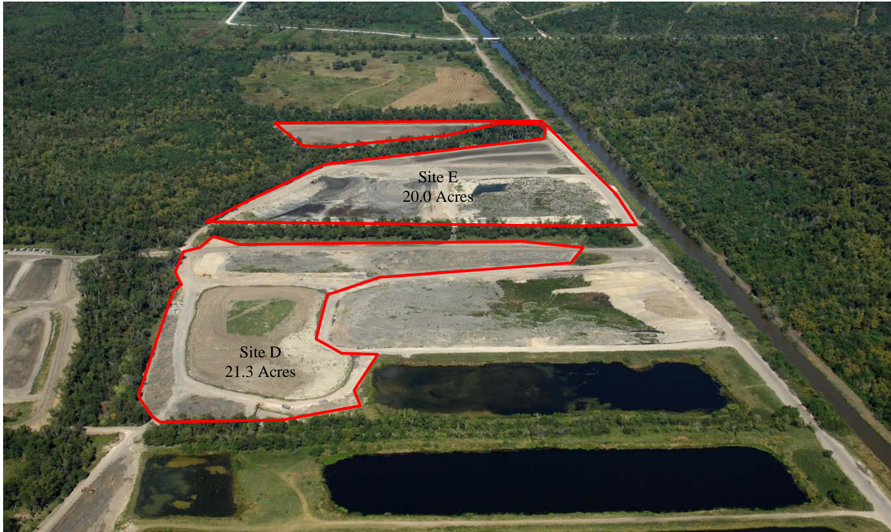
Figure 12. Aerial View of Sites D and E at Walker Road Soil Mixing Area
