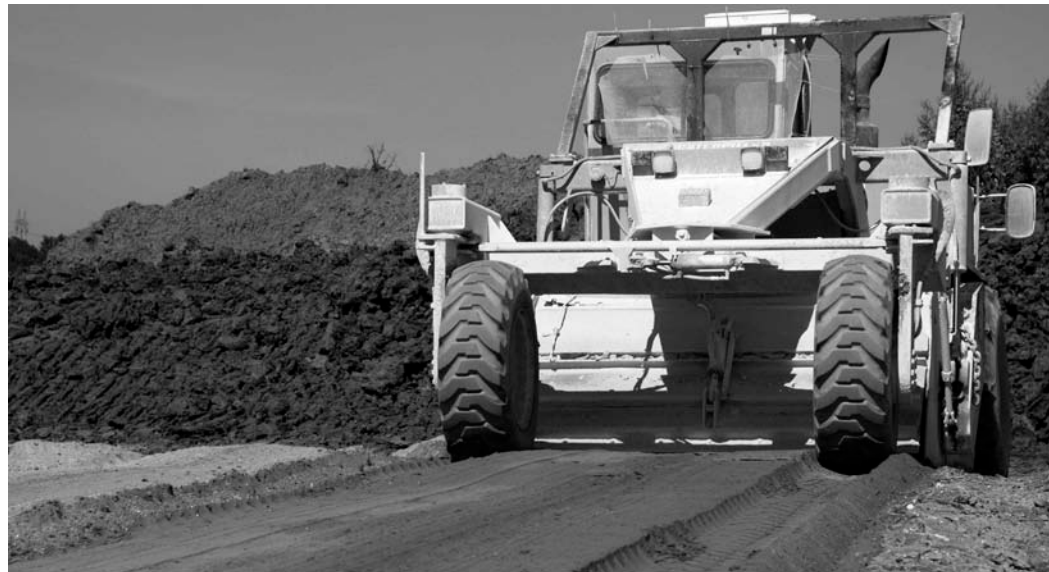
Figure 16. High Speed Pulverizer
