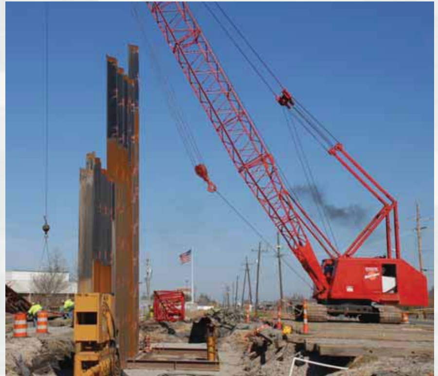
Construction of concrete floodwalls will require pile driving.
