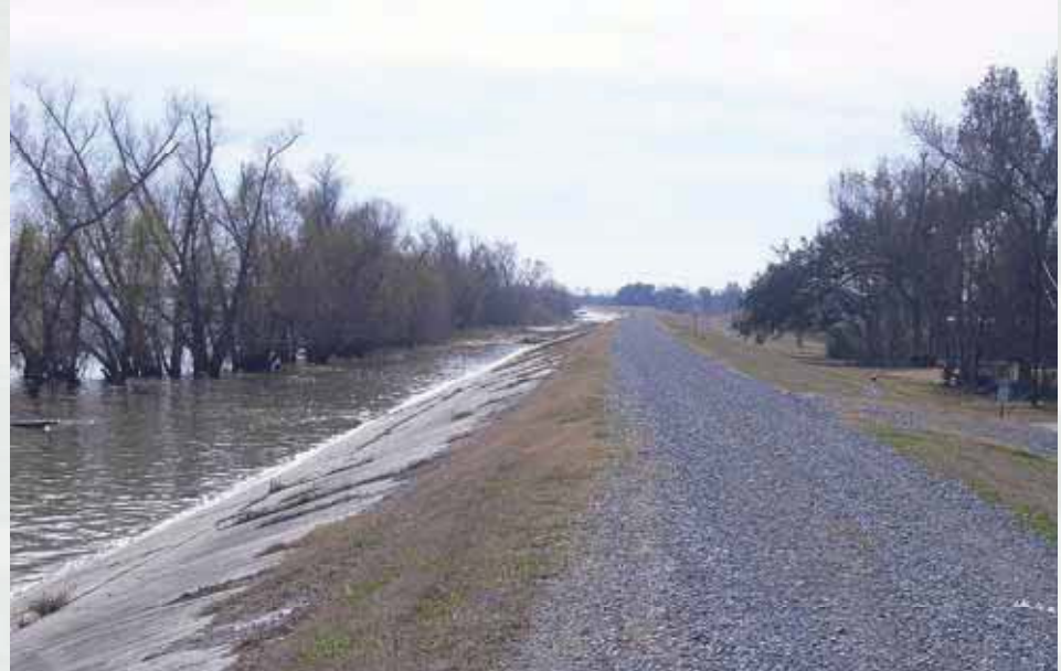
Many Mississippi River levee stretches include gravel topped crowns and concrete slope paving on the flood side.
