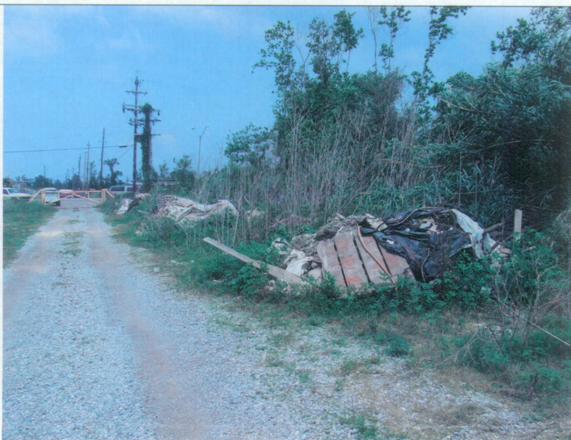
Photo #: 4 of 7 Time: 1252 Description: N 30.01062 W 89.94978; Multiple piles of C&D, Concrete, Asphalt
