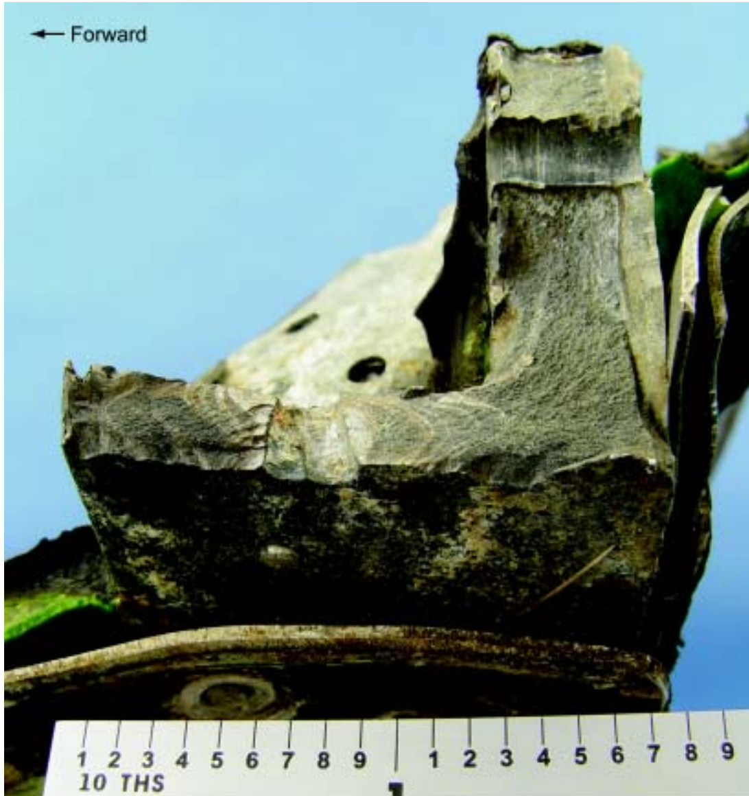
Figure 6. Right Wing Rear Spar Lower Spar Cap Fracture
