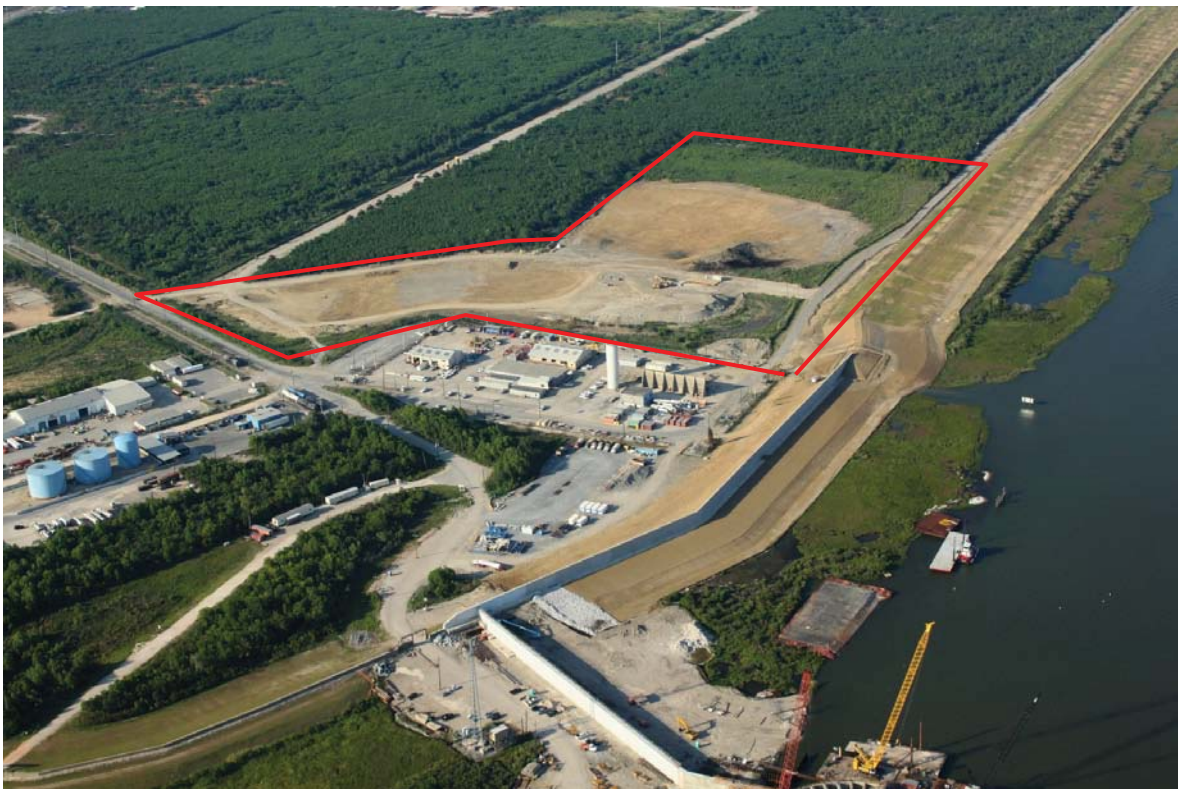
Figure 4. Aerial photograph showing vegetative clearing and placement of REM (outlined in red) on 22.41 acres of BLH in and around Stumpf Borrow Site as of 6 July 2011.
