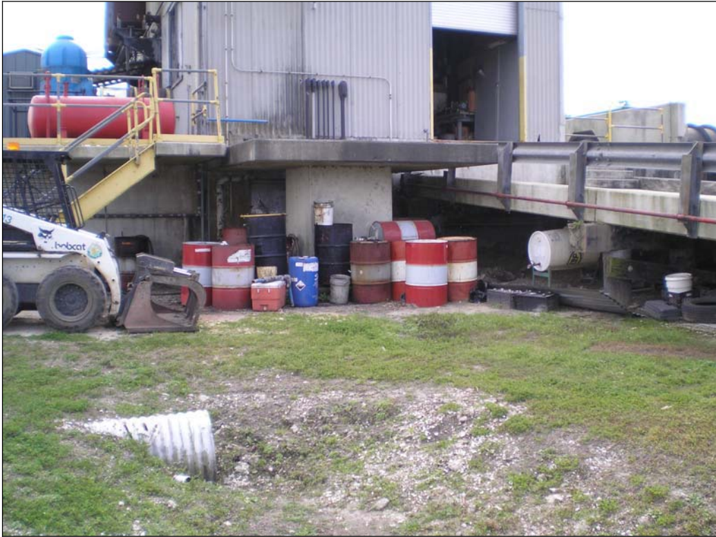
Photograph 11. Oil drums and other materials stored adjacent to pump building
