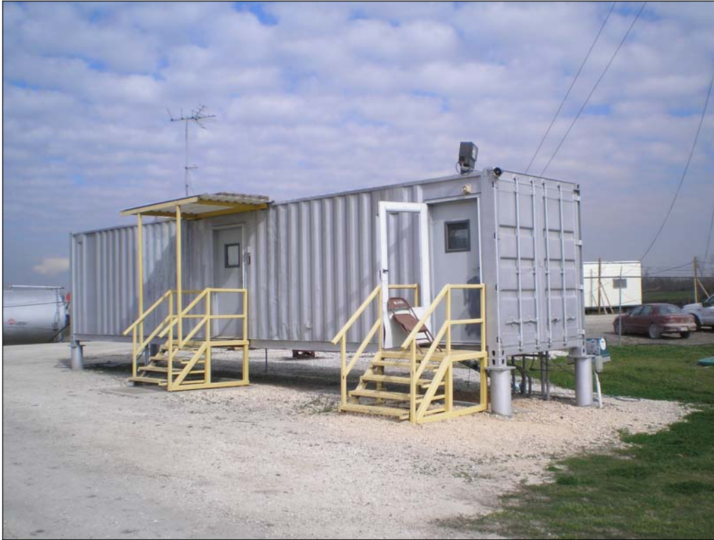
Photograph 9. Office/control trailer on subject property
