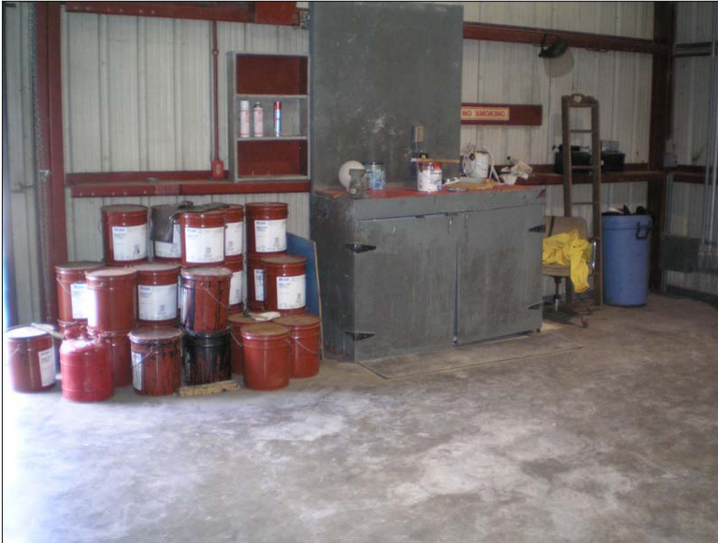
Photograph 1. Oil and paint containers stored inside pump station
