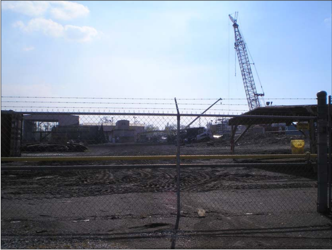
Photograph 21. Shipyard on property southwest of pump station
