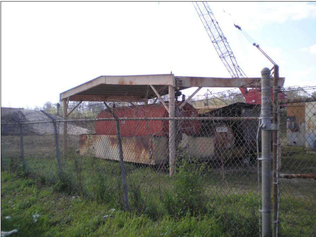
Photograph 20. Abandoned fuel tanks on property southwest of pump station
