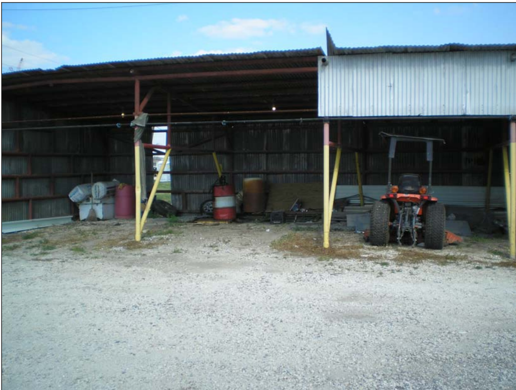
Photograph 6. Maintenance shed with mowers and gasoline storage
