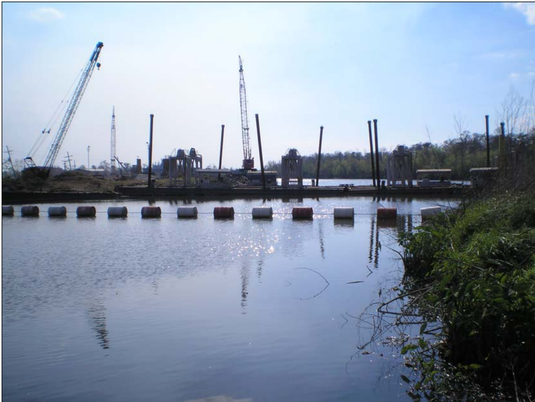
Photograph 16. Discharge basin west of pump station, view to the west
