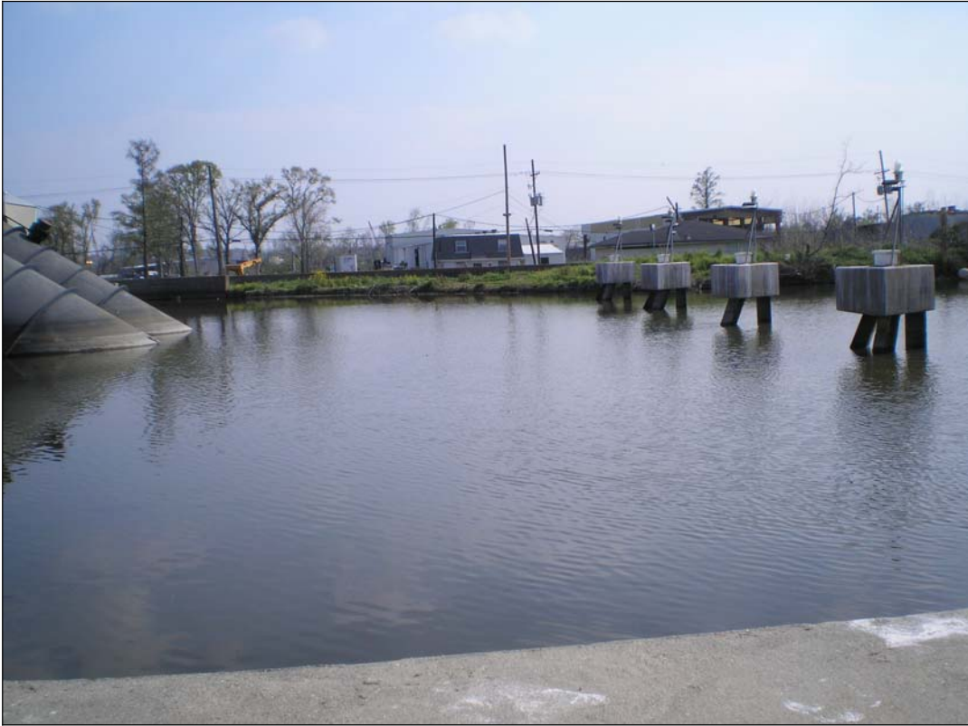
Photograph 17. Discharge basin west of pump station, view to the south
