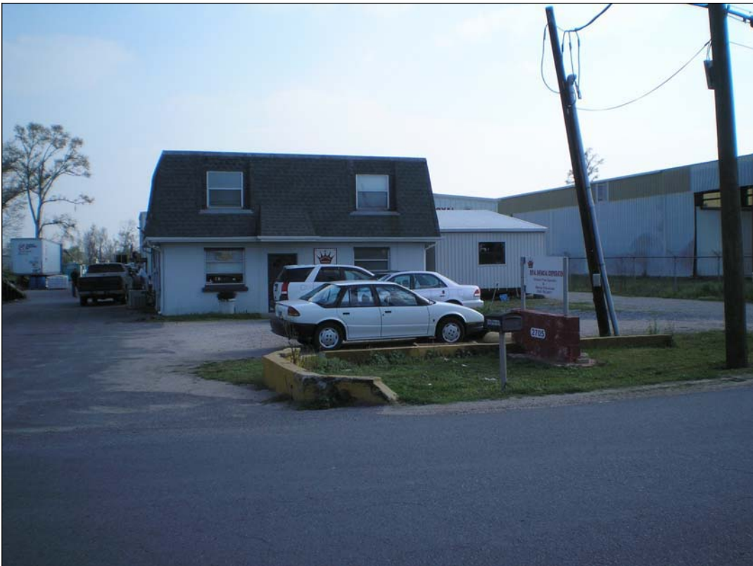
Photograph 18. Adjacent property south of pump station
