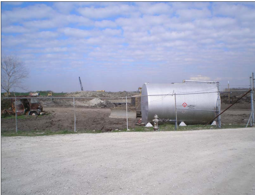
Photograph 8. Diesel storage tanks on adjacent levee construction site to the west
