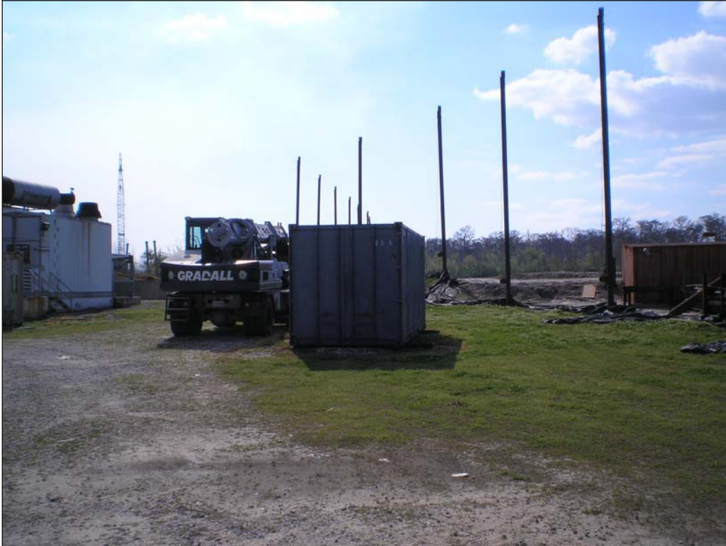
Photograph 10. Storage box and crane on subject property
