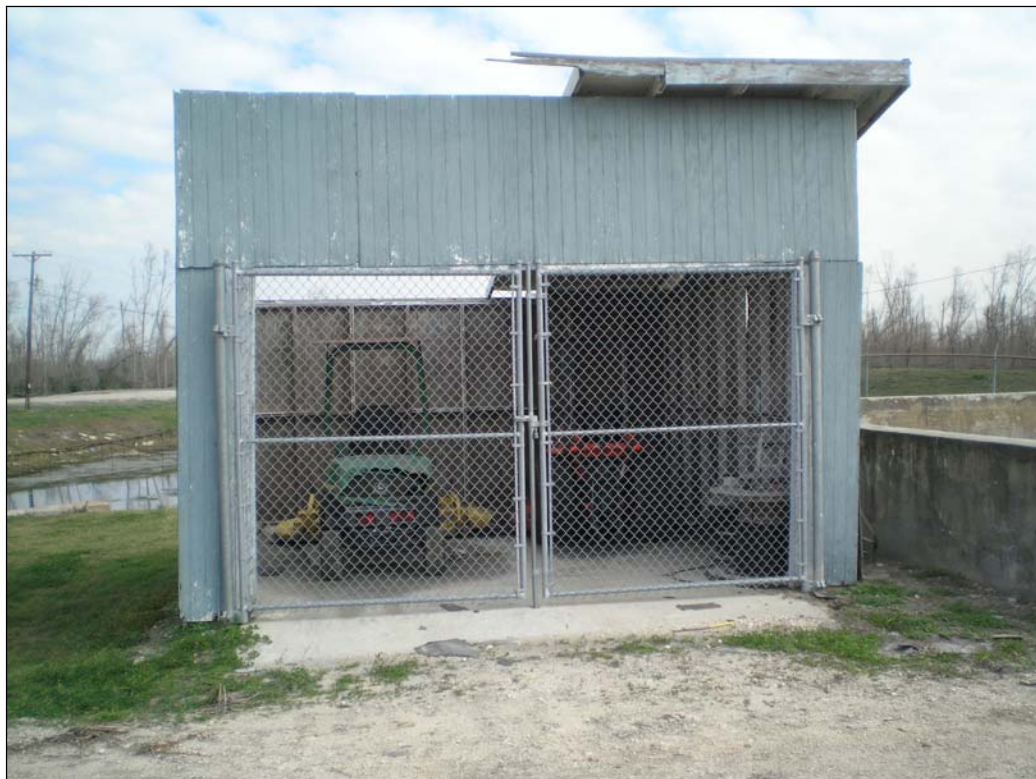
Photograph 10. Equipment storage shed on subject property
