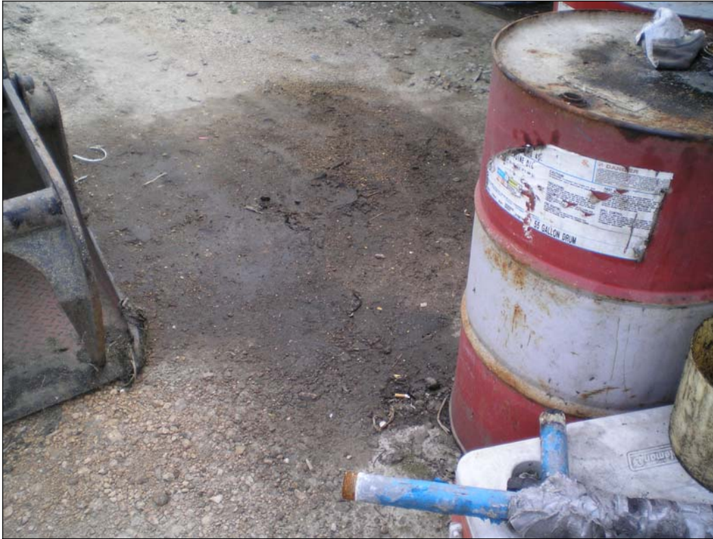
Photograph 13. Oil/fuel spill adjacent to stored barrels near pump building
