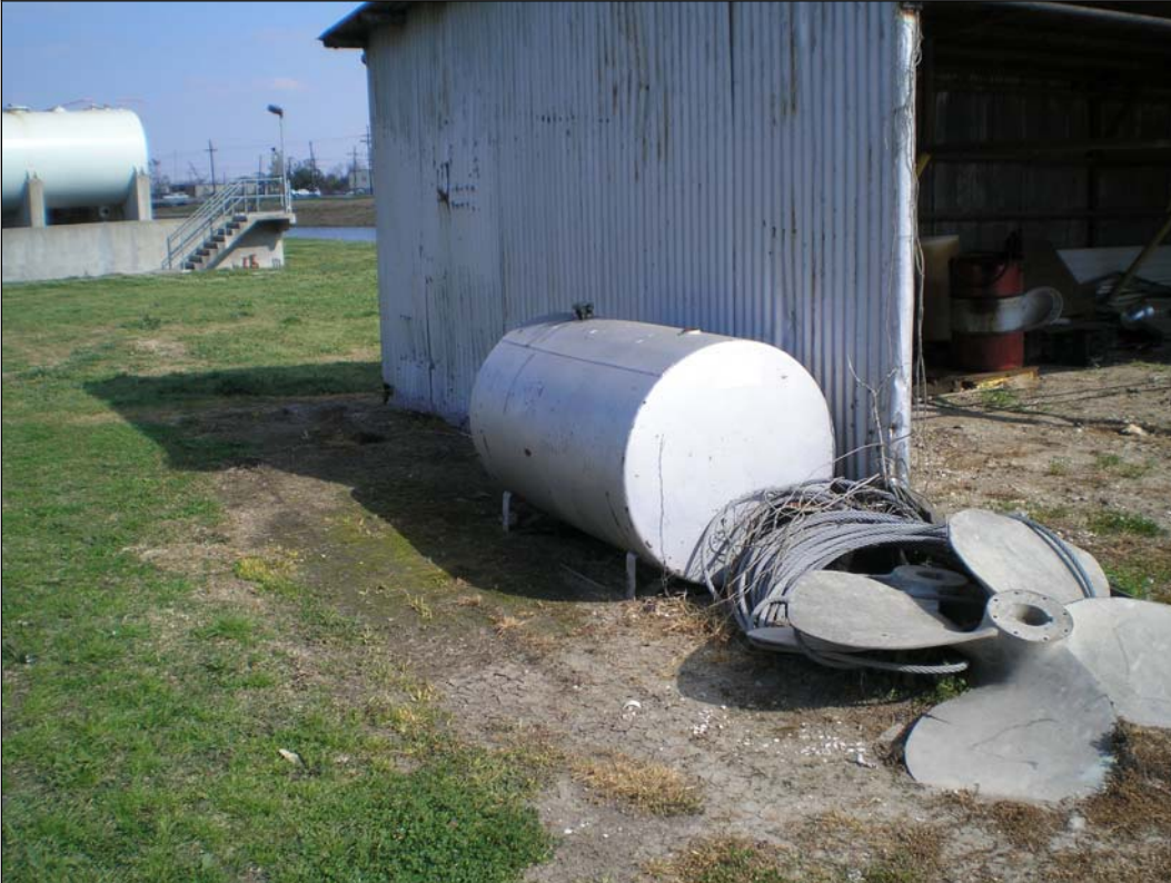
Photograph 8. Waste oil tank adjacent to maintenance shed
