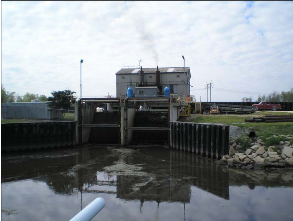
Photograph 1. New pump station, view to the south
