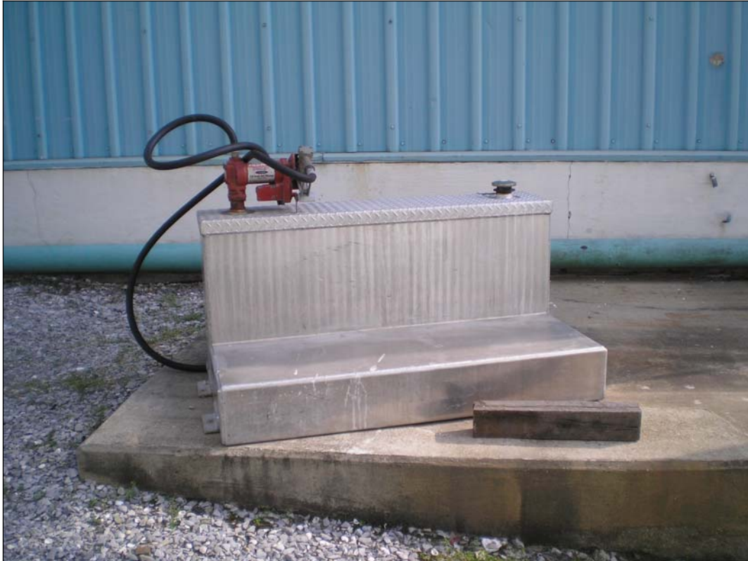
Photograph 15. Diesel truck tank adjacent to pump station building
