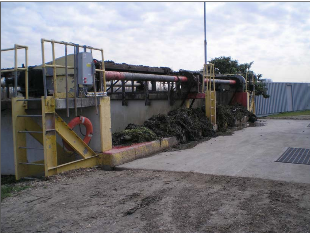
Photograph 18. Debris raked from intake pond at pump station
