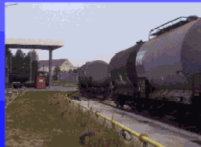
Fuel transfer terminal with spill apron
