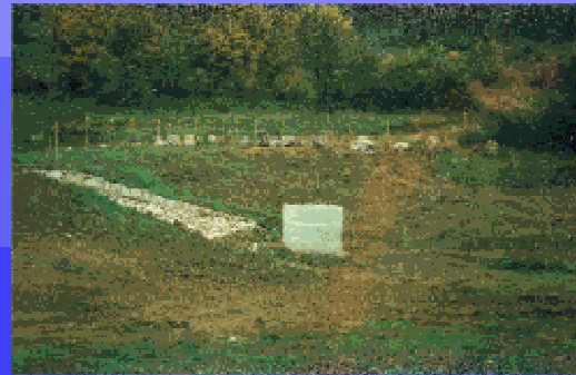
Check Dam at Hohenfels Training Area
